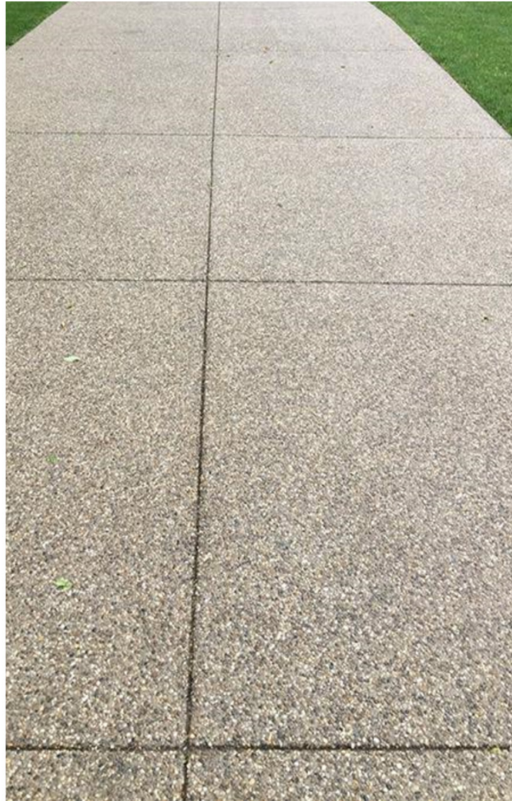
Monolithic concrete paving
