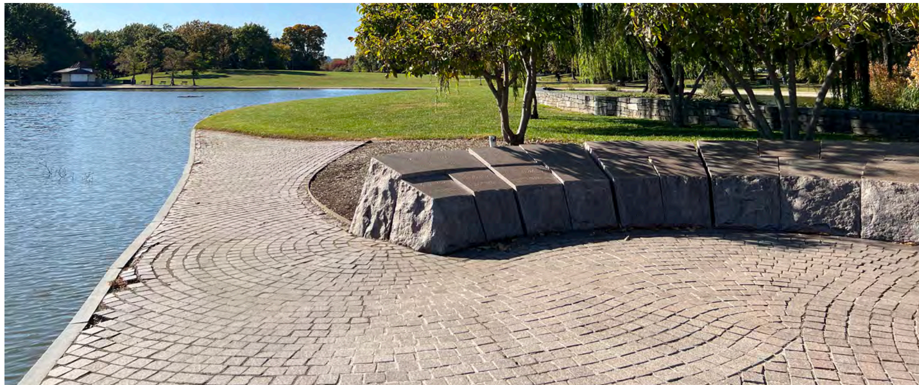
SIGNERS ISLAND | EXISTING COBBLESTONE
