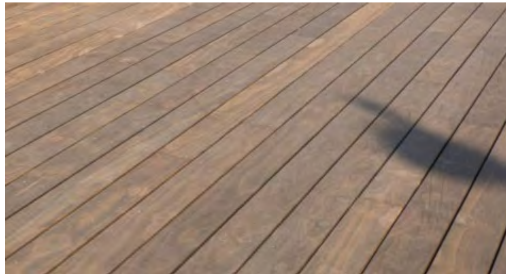
WOOD DECKING AT LAKE RING -KEBONY
