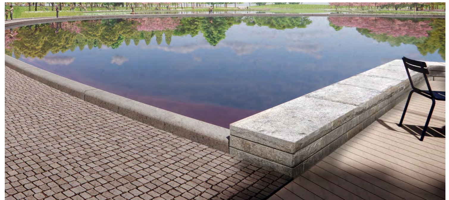
LAKE RING COBBLE PAVING, CURB, STACK STONE WALL AND DECKING
