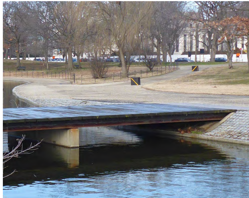
EXISTING, NON-ADA COMPLIANT BRIDGE
