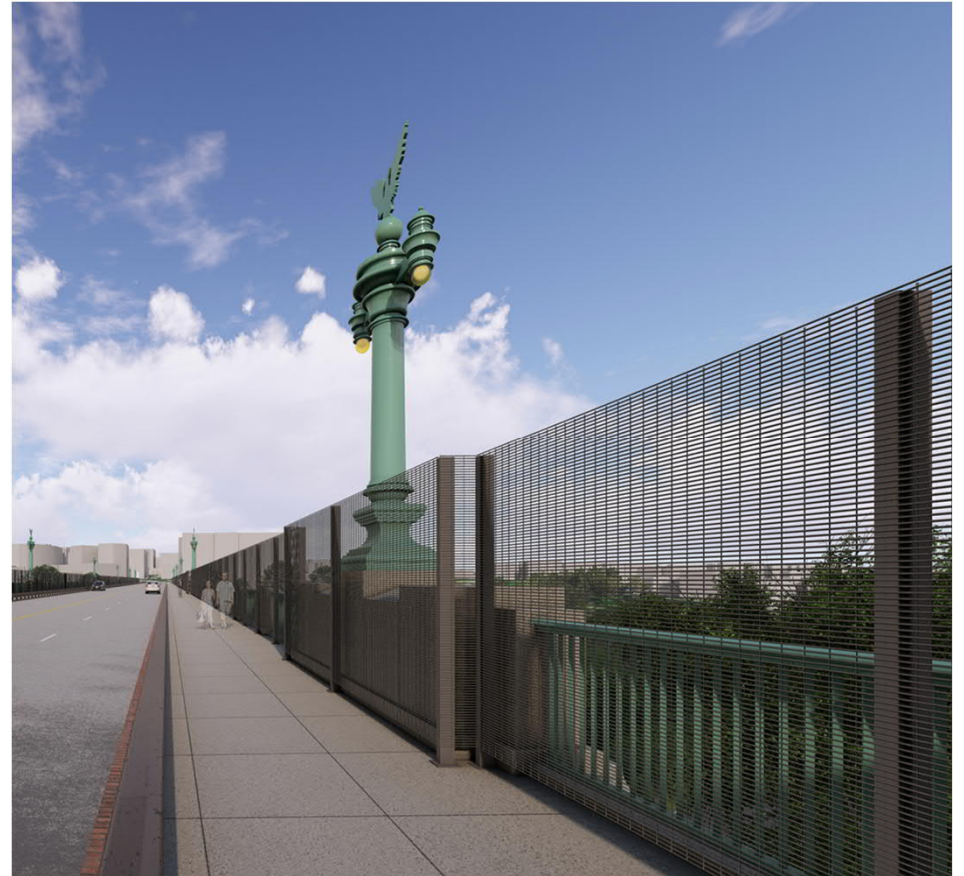
Option 2 Wire Mesh Addition ( Further considered by CFA )
