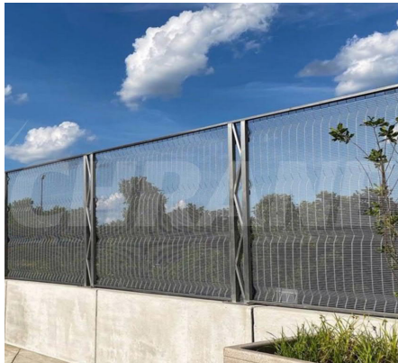
Reference Photo of Bridge 341
