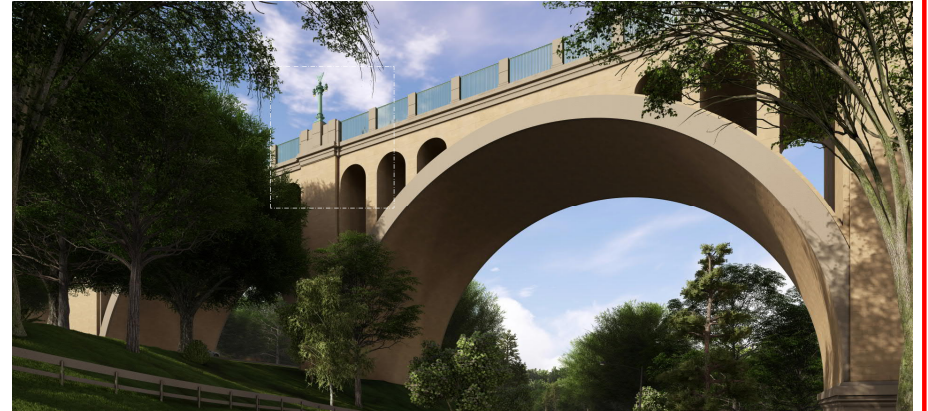
View from Rock Creek Park with Single Light Pole Condition
