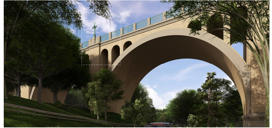
View from Rock Creek Park with Single Light Pole Condition
