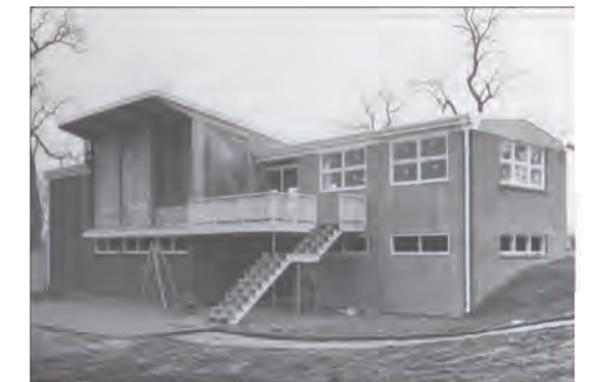
Existing Clubhouse under construction, 1964
