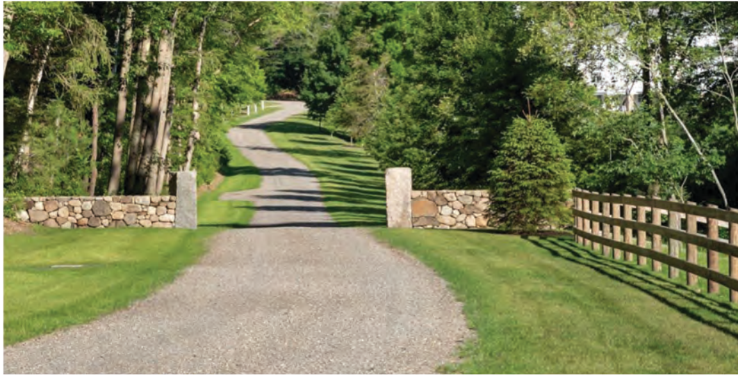
Crushed Stone Paving
