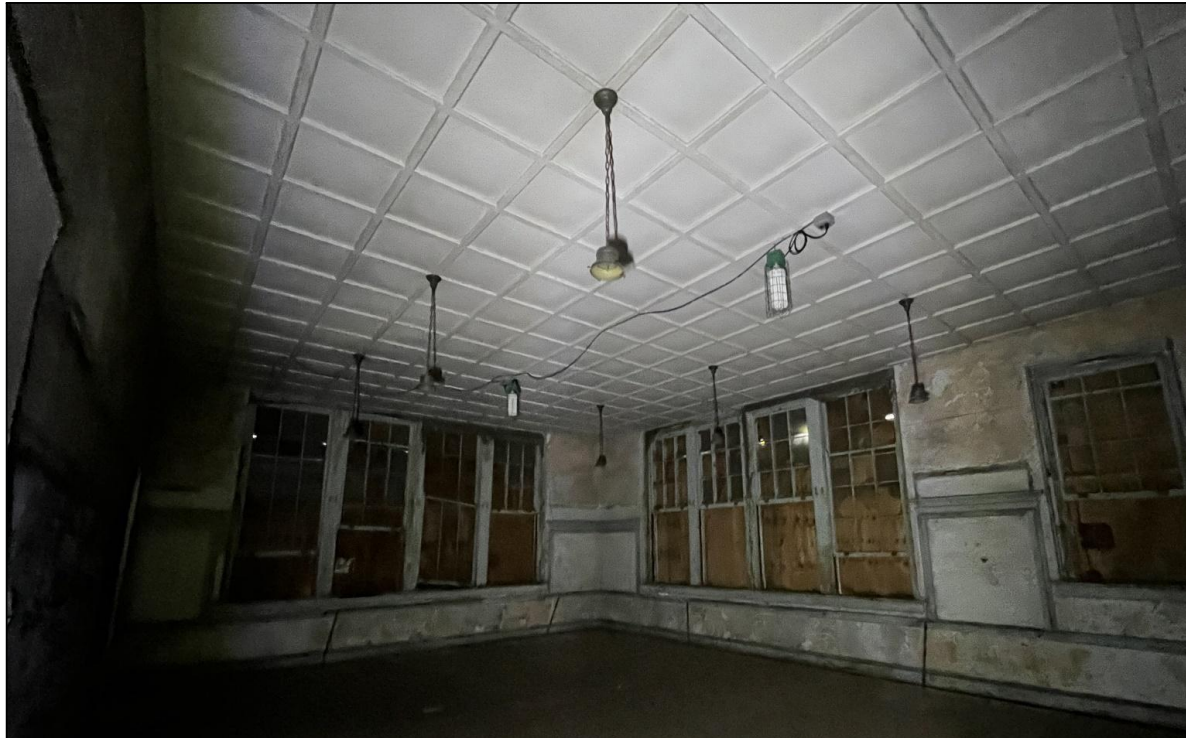
Figure 7: Second floor classroom, note intact ceiling.
