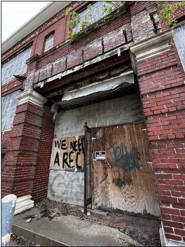
Figure 3: Entrance on north elevation.
