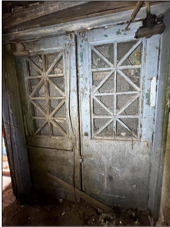
Figure 5: Wooden door at northern entrance.
