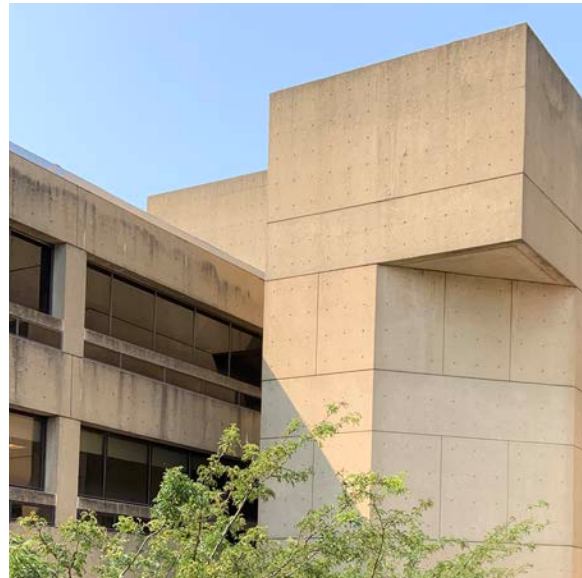
PRECAST CONCRETE [UDC CAMPUS]
