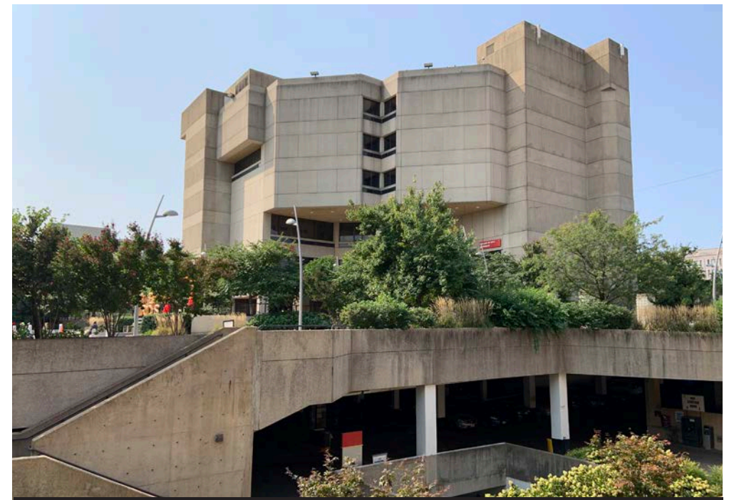
5 | View from Adjacent Building Looking SW
