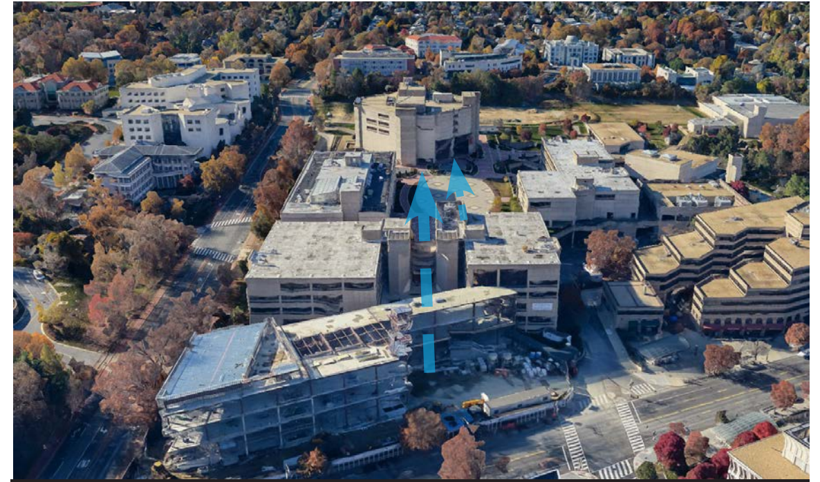
4 | Aerial View Looking West
