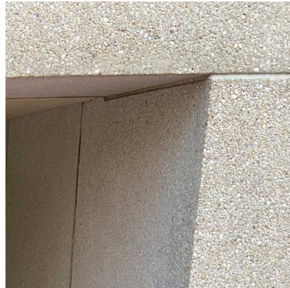
PRECAST CONCRETE [UDC CAMPUS]
