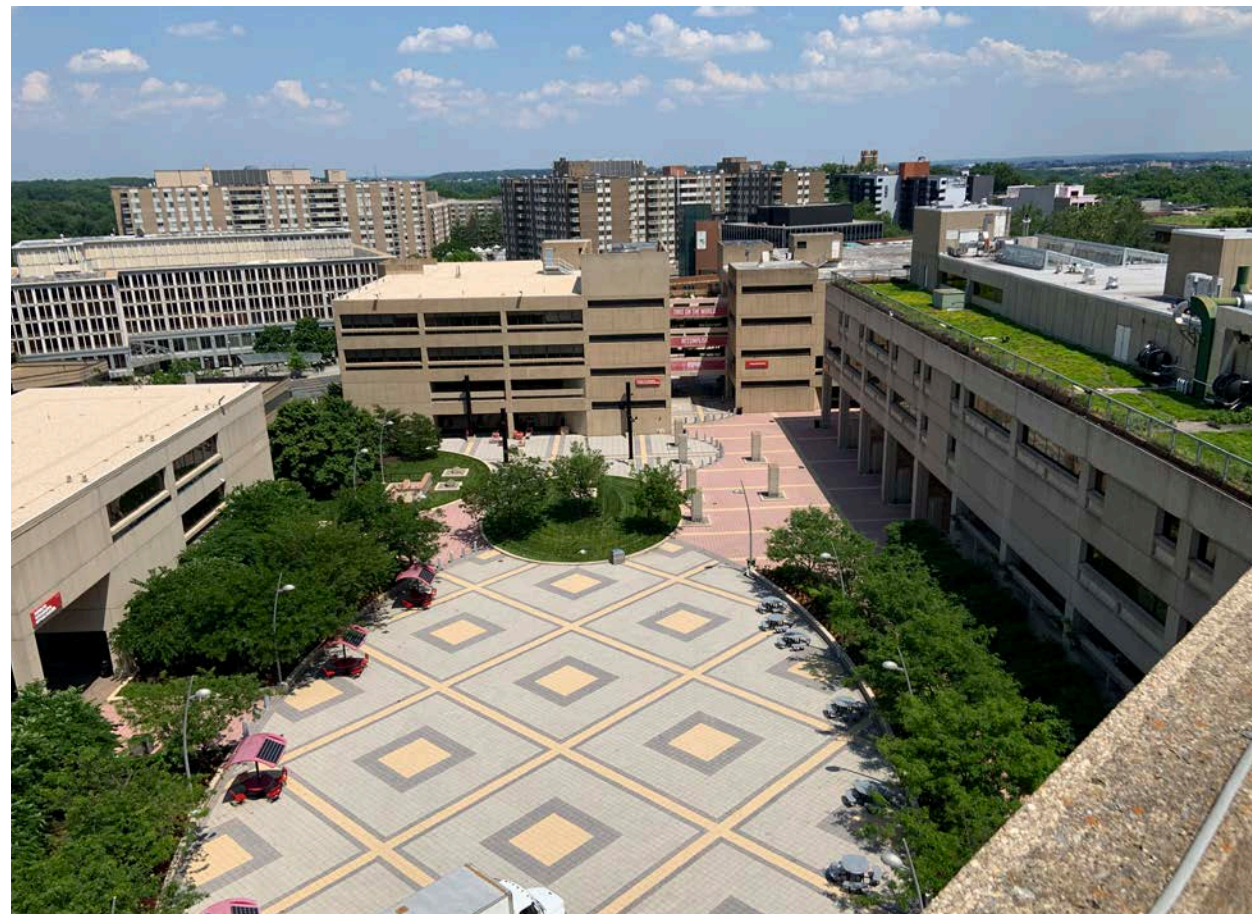
1 | View from Building 41 Roof Looking East
