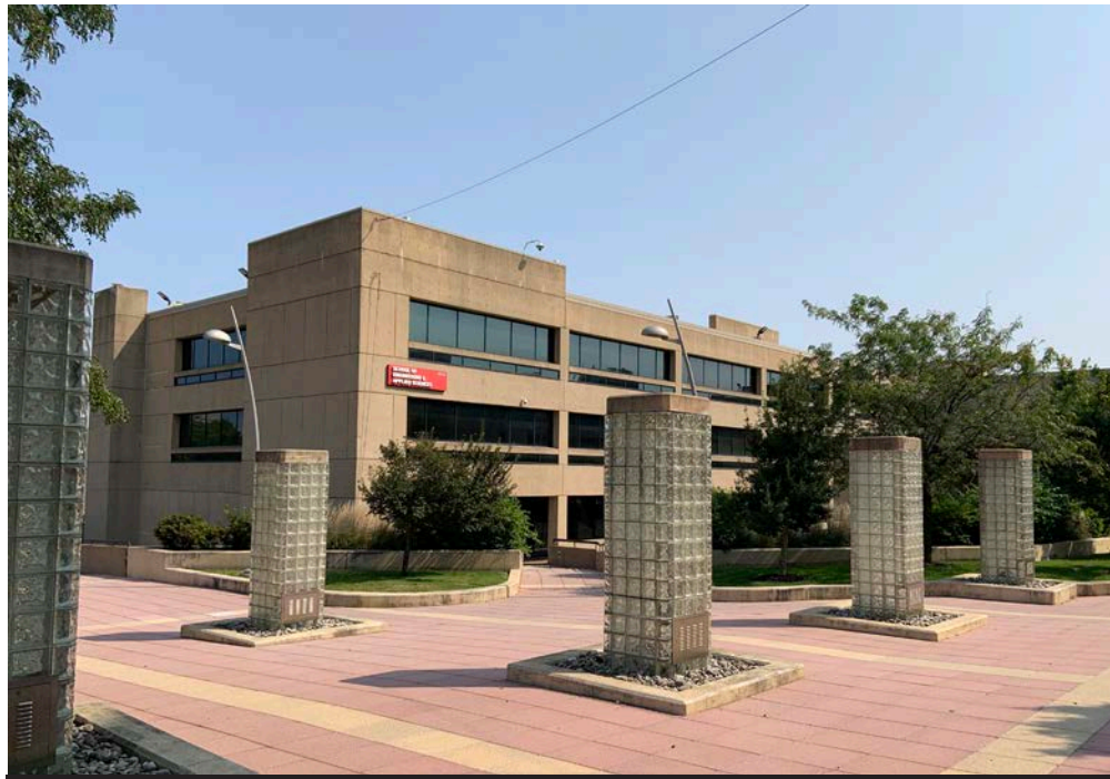
3 | View of Building 32/42 Looking East
