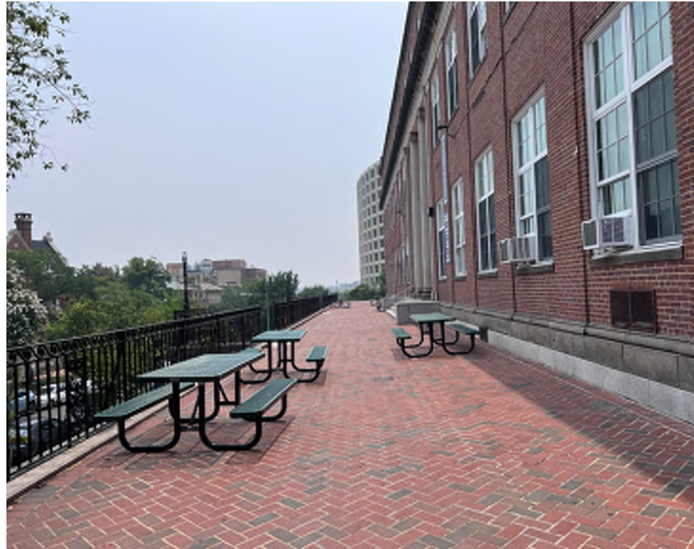
VIEW FROM VERANDA
