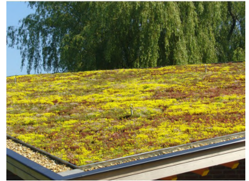
Green Roof Sedum
