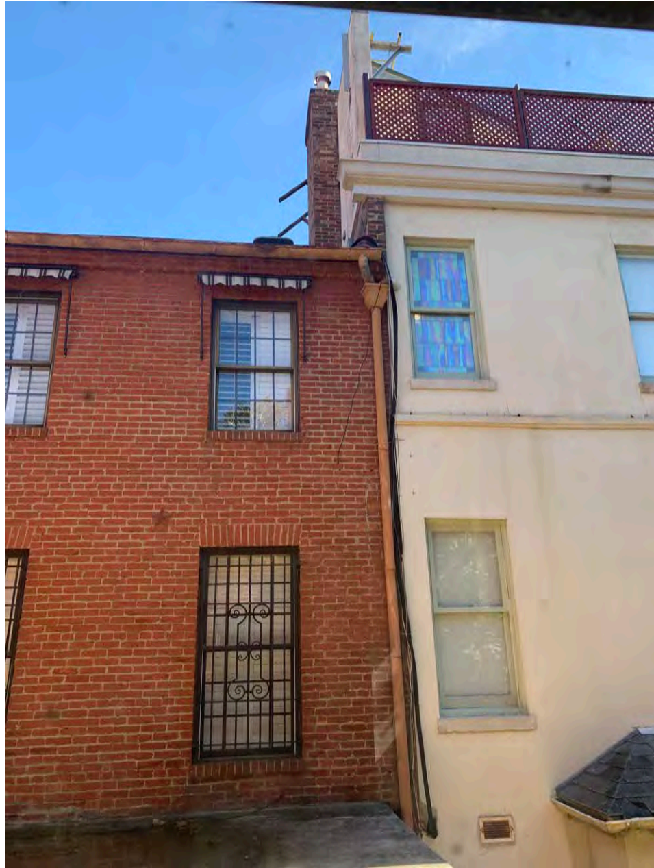
West Side of 1132 29th Street NW
