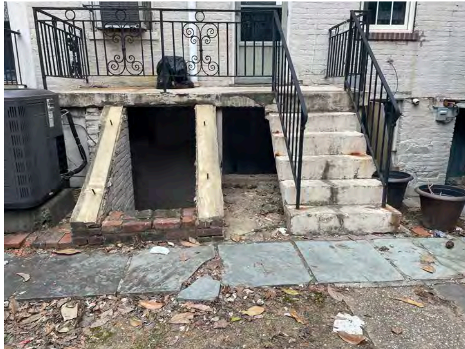
Existing Rear Sub Basement at 2912 M Street, Door Proposed to be removed and inset brick to fill in opening
