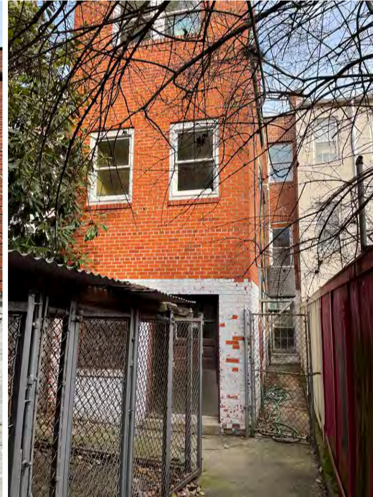
East and South Elevations of the two-story rear addition (c.1963 – 1960's) show the delineation between the historic rear elevation and the newer construction.
