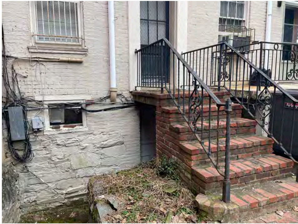
Existing Rear Sub Basement at 2914 M Street, Door Proposed to be Removed and Inset Brick to Fill in Opening
