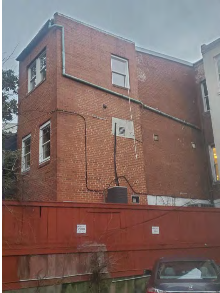
East and South Elevations of the two-story rear addition (c.1963 – 1960's) show the delineation between the historic rear elevation and the newer construction.
