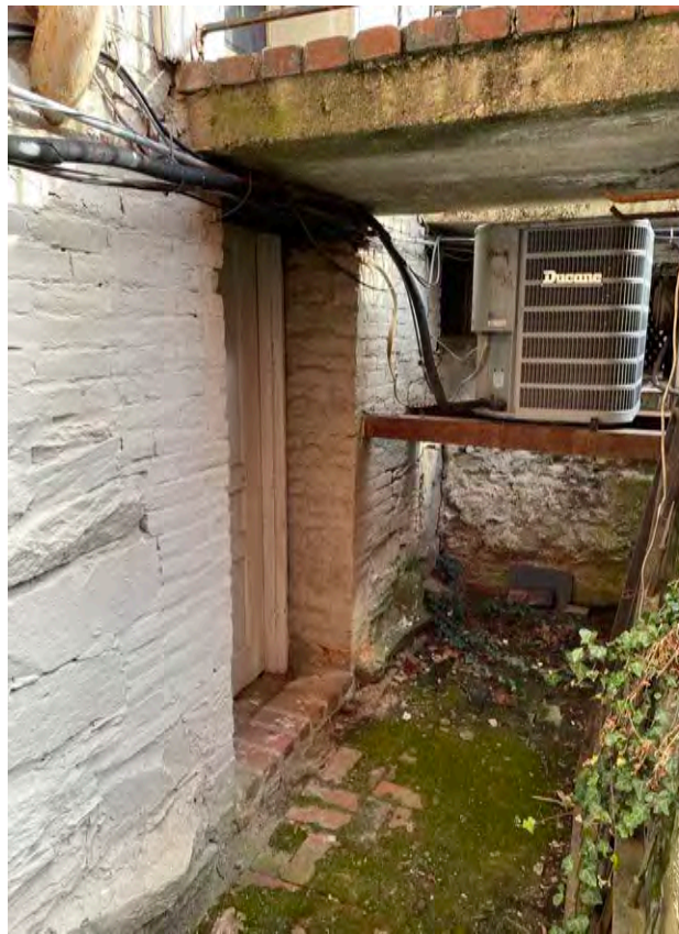
Existing Rear Sub Basement at 2914 M Street, Door Proposed to be Removed and Inset Brick to Fill in Opening
