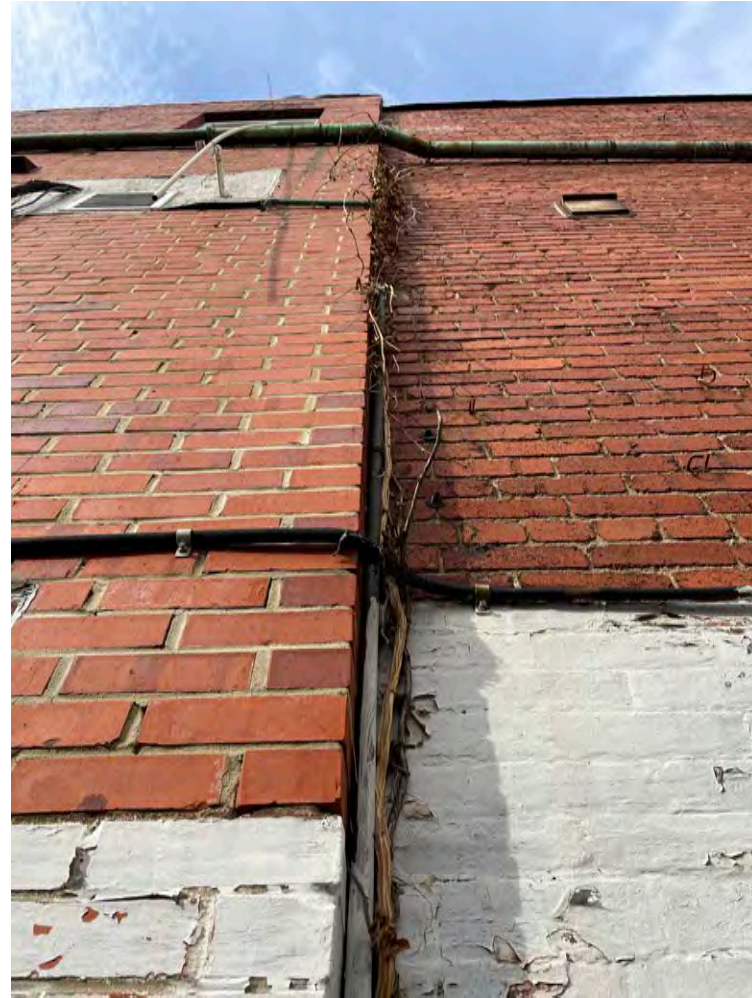
East and South Elevations of the two-story rear addition (c.1963 – 1960's) show the delineation between the historic rear elevation and the newer construction.
