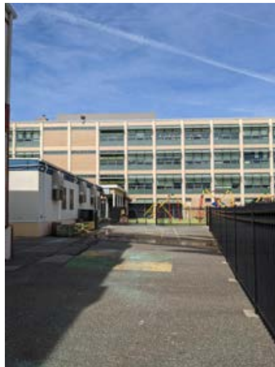
SOUTH -MAIN BUILDING
