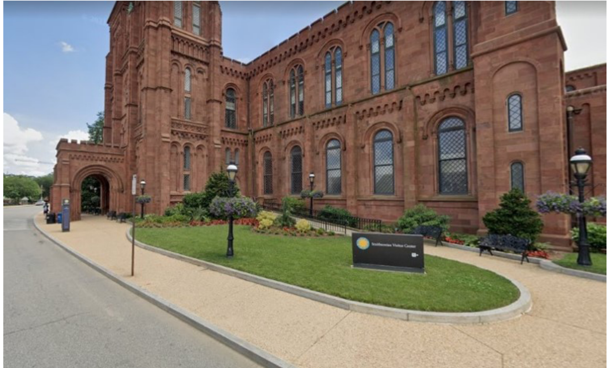
Figure 3.3.6.a – Existing west accessible ramp to the Castle's North Tower
