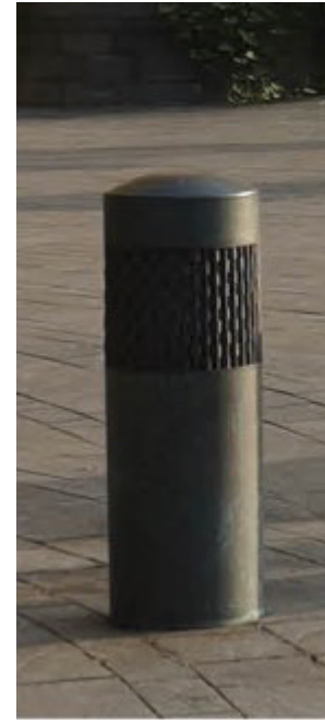
Figure 3.3.2.d – Bollard mock-up at the porte cochere, for Consulting Parties review; example of bronze bollard cover at National Museum of the American Indian
