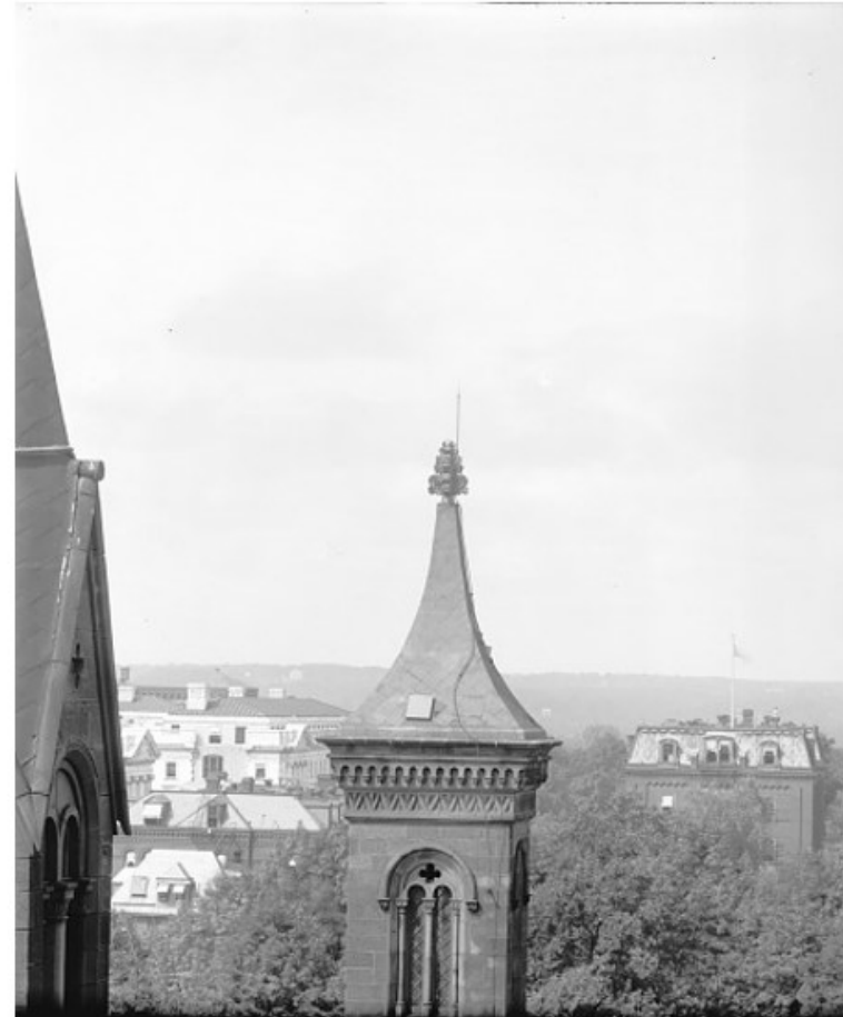
Figure 3.4.6.a – Historic image c.1930 of the West Tower with lightning protection
