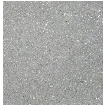
(B) – Stair - Poured in-place concrete with architectural finish
