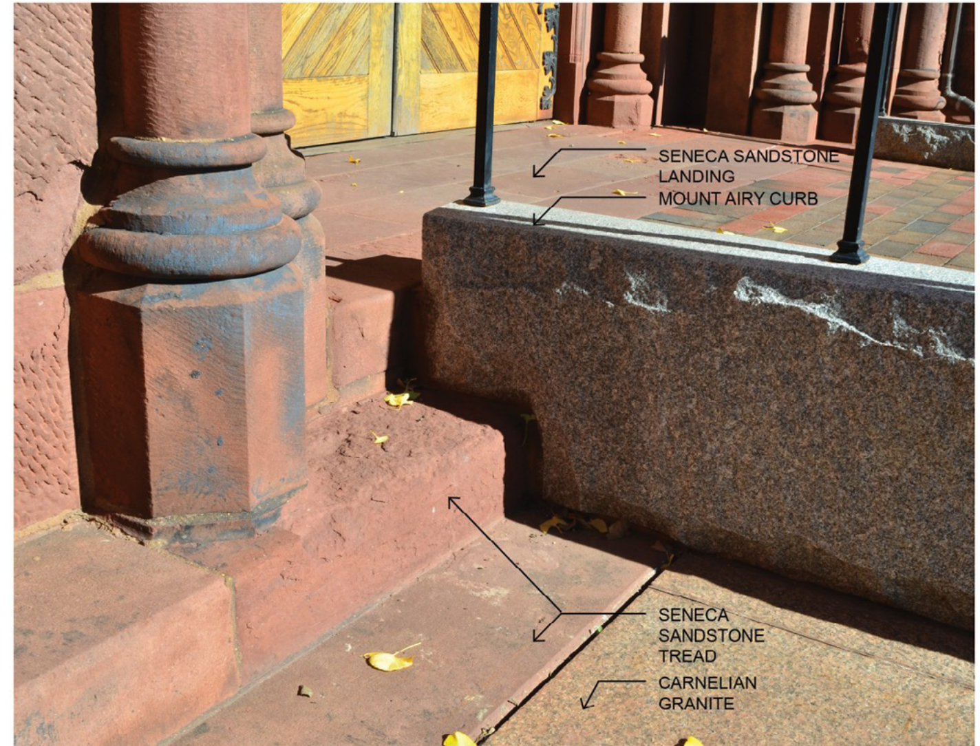
Figure 3.3.5.b – Existing ramp connection to the historic sandstone stair treads
