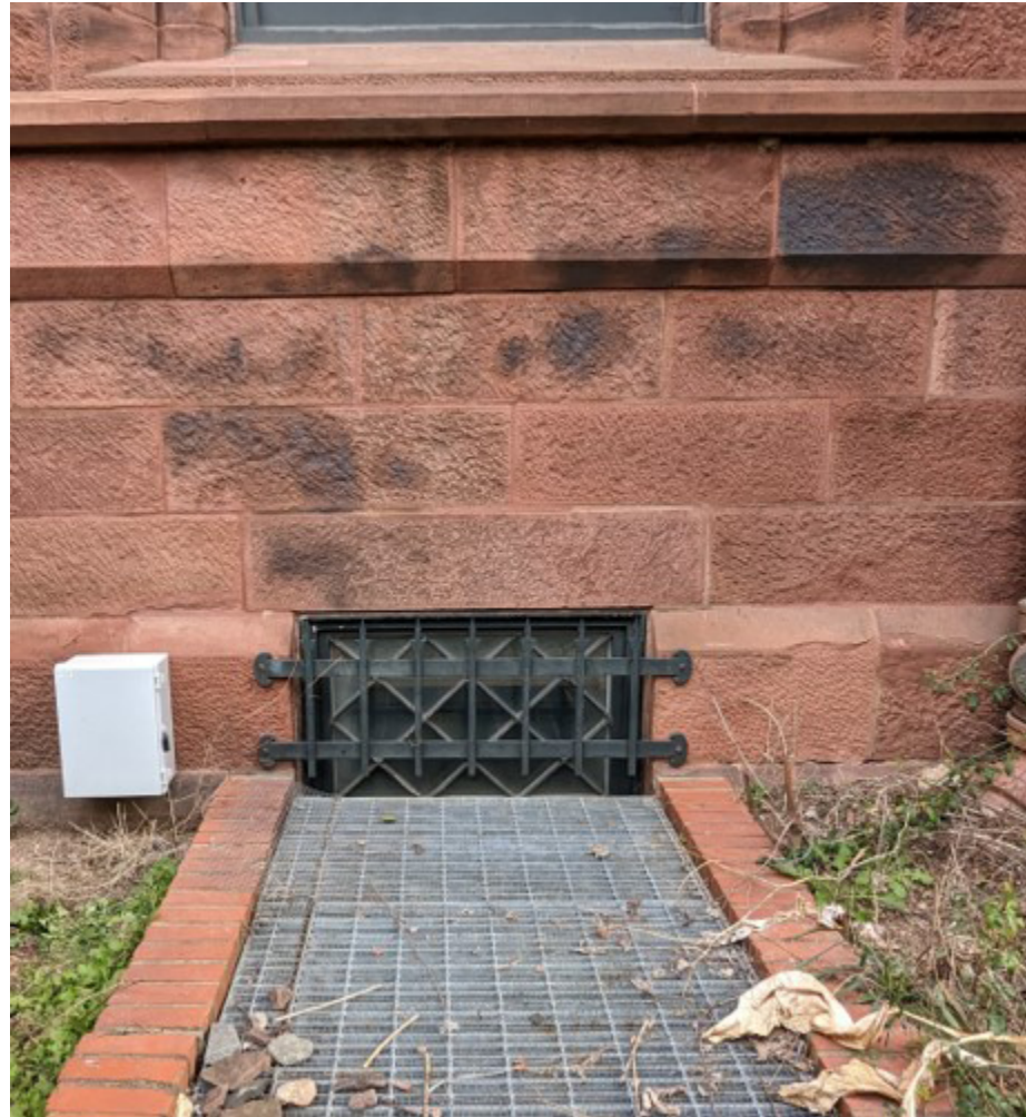
Figure 3.5.3.a - Photograph of existing basement window at the southeast side of the Main Building; note the metal window security grille
