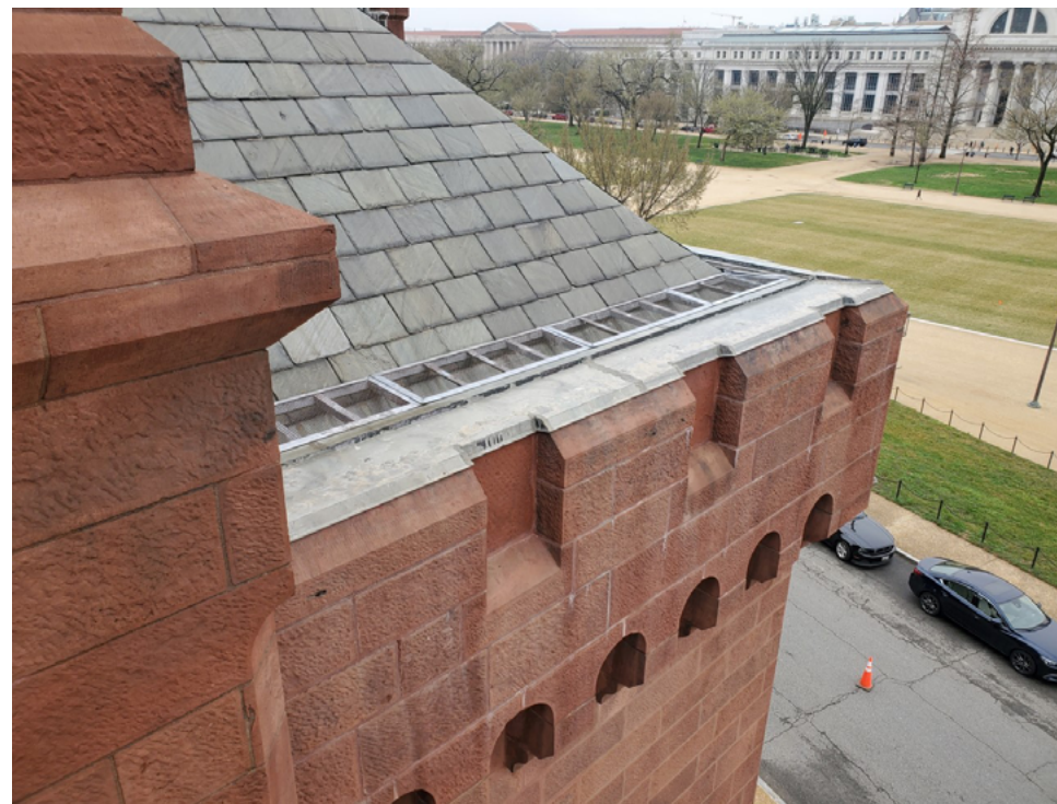
Figure 3.4.2.c – Typical condition of slate roofing shingles
