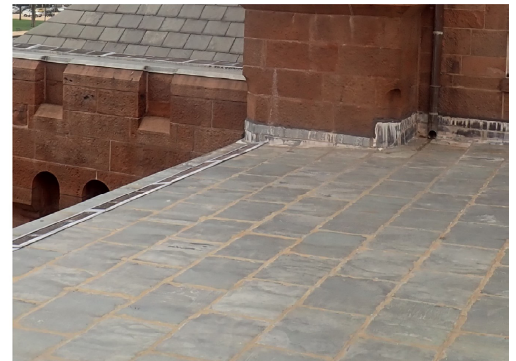
Figure 3.4.2.d – Typical condition of flat seamed lead coated copper roofing
