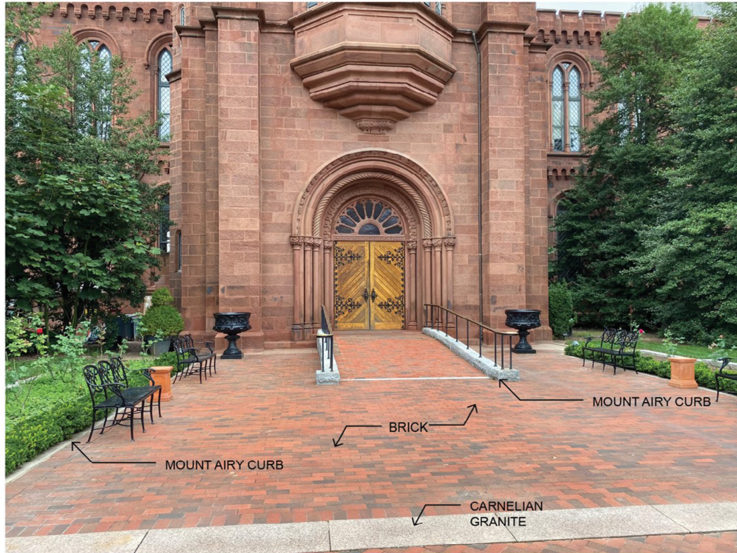
Figure 3.3.5.a – Existing South Entrance condition
