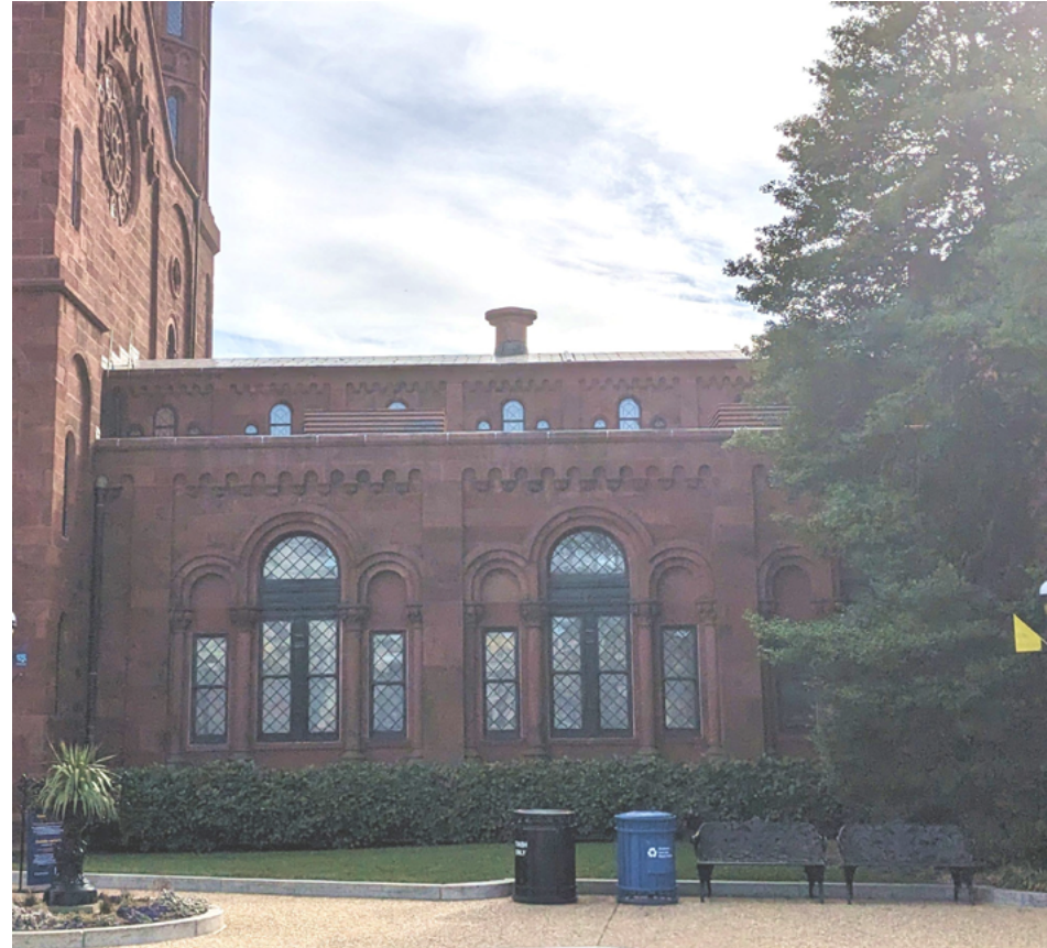
Figure 3.4.4.c – West range existing mechanical penthouses
