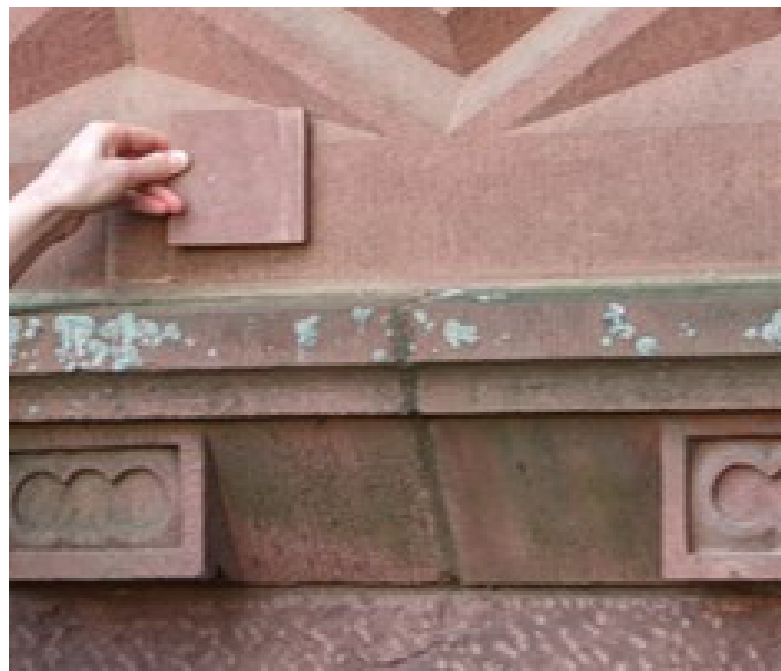
Figure 3.5.2.a - St. Bees sandstone, replacement stone where existing sandstone cannot be reused
