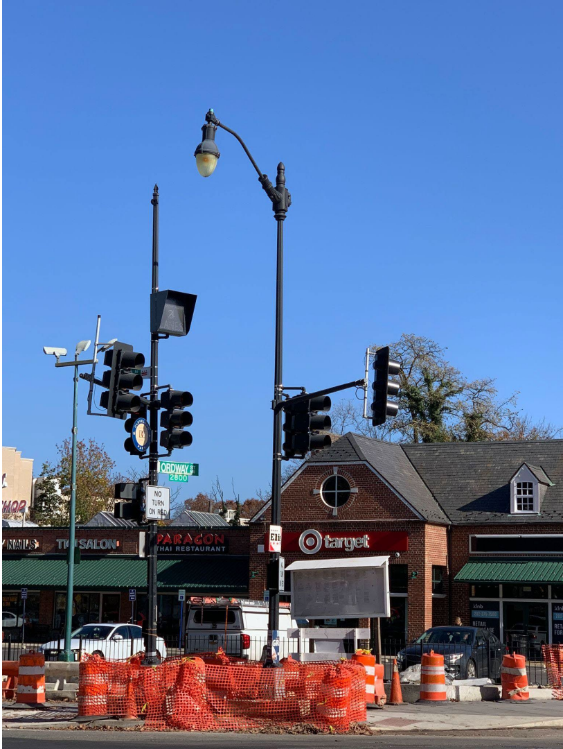
9. Connecticut & Ordway (tall post on NE corner)
