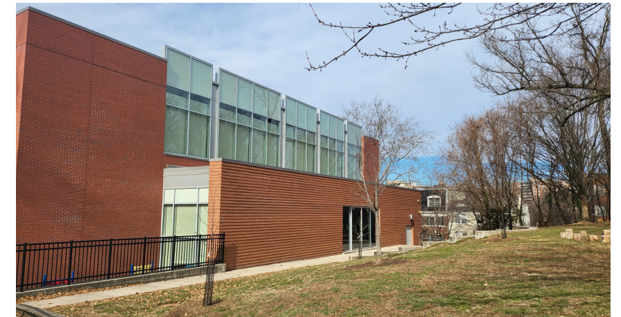
08: Detail view of East façade
