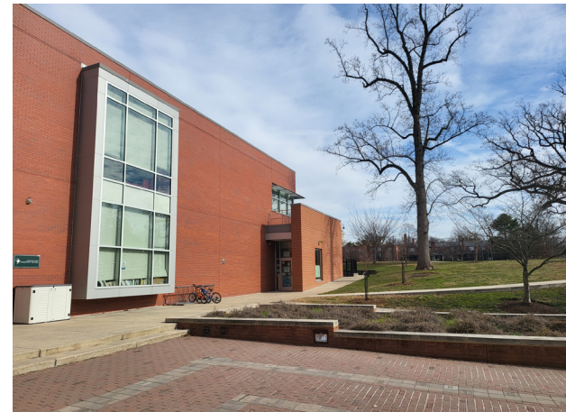
07: Detail view of South façade
