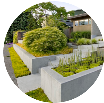
Cast-In-Place Concrete Walls
