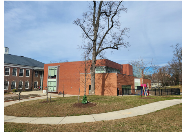
03: South-East corner of Existing Building
