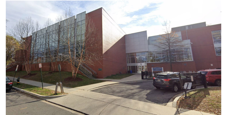
02: Service Entrance view from Davis Place
