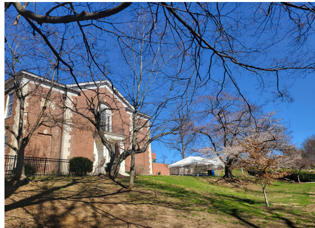
05: South façade of Historic building
