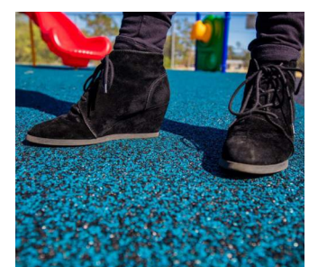
5 Poured In Place Rubber Play Surface
