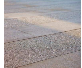
2 Exposed Aggregate Concrete Detailing
