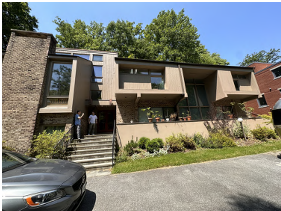
4. VIEW FROM THE DRIVEWAY TO THE FRONT OF THE HOUSE.
