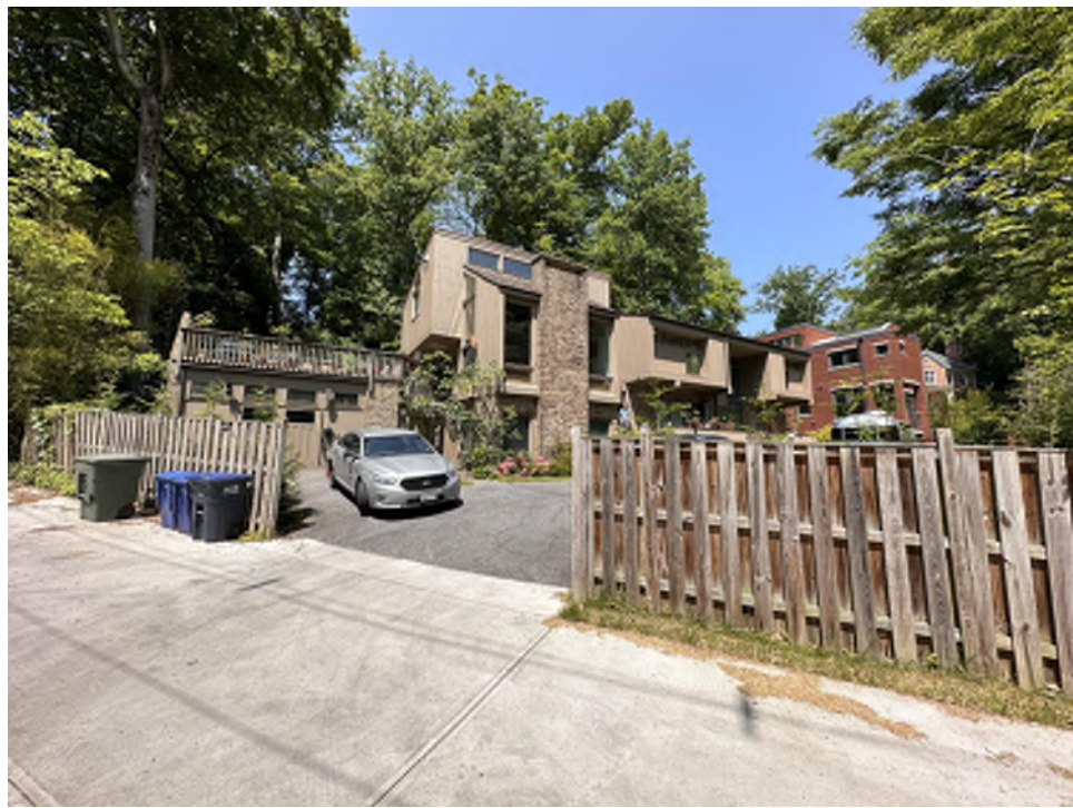
2. DRIVEWAY VIEW FROM THE ALLEY.
