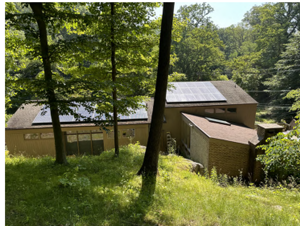
4. REAR YARD AND REAR FACADE
