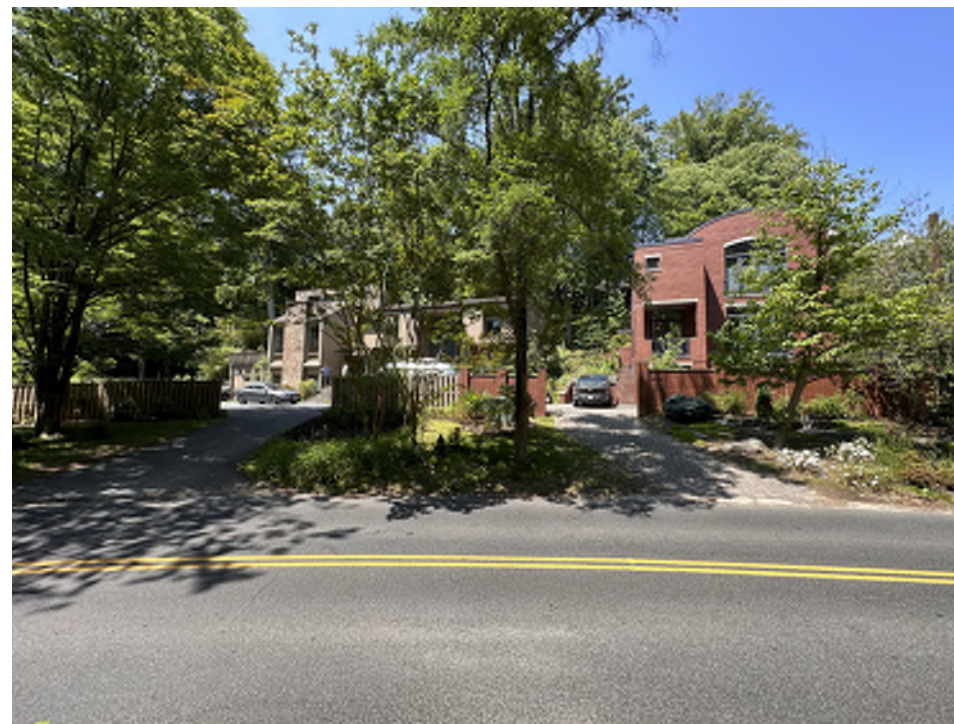
3. VIEW FROM ACROSS BROAD BRANCH RD NW.
