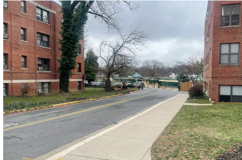
2 West Curb on MacArthur Blvd
