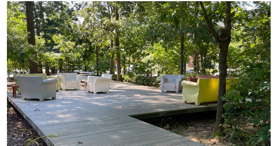
The metal decking would offer a permeable surface that would enable the retention of trees.
