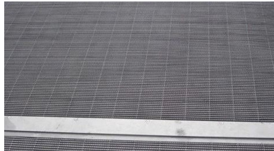
The metal decking material comes in multiple formats, including one that would accommodate high-heeled footwear and is slip-resistant.
