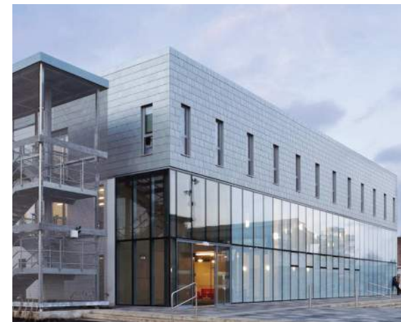
GLAZING: Metal Mesh Inner Layer Increased Privacy + Controlling Views, Light Diffusion
