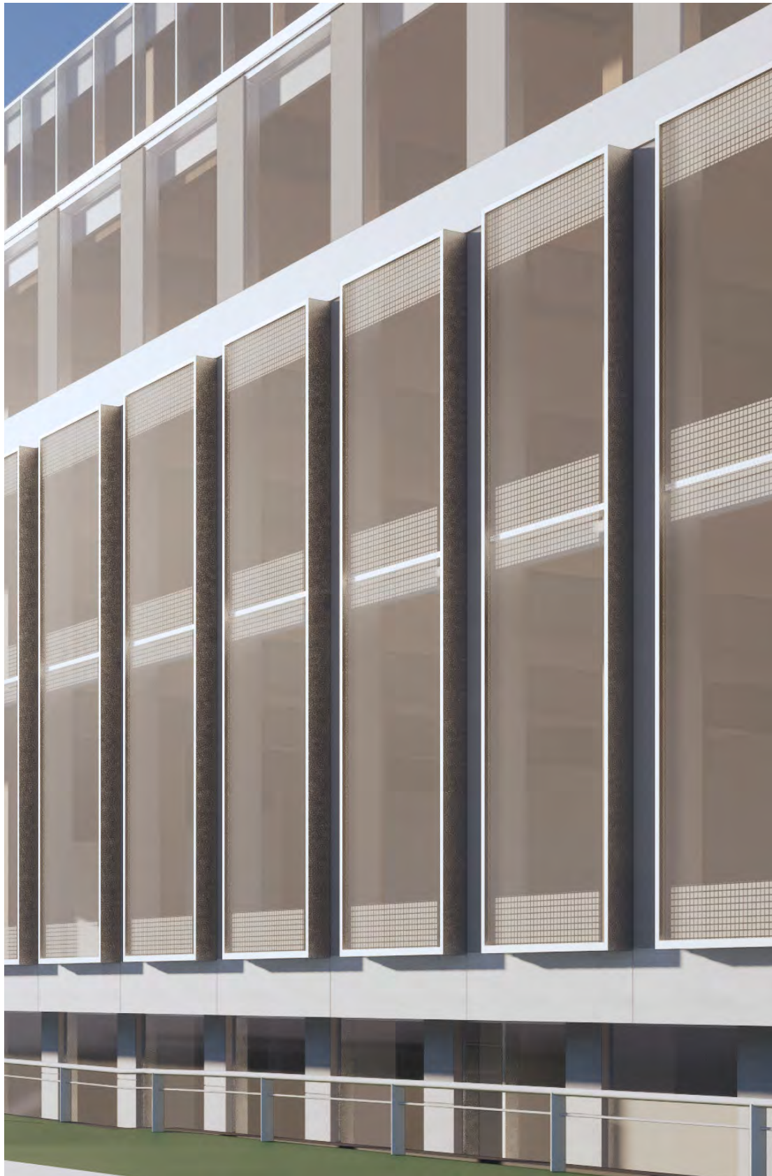
FRB-EAST ADDITION BAYS PROJECT 14" FROM FACE OF ADJACENT GLAZING
