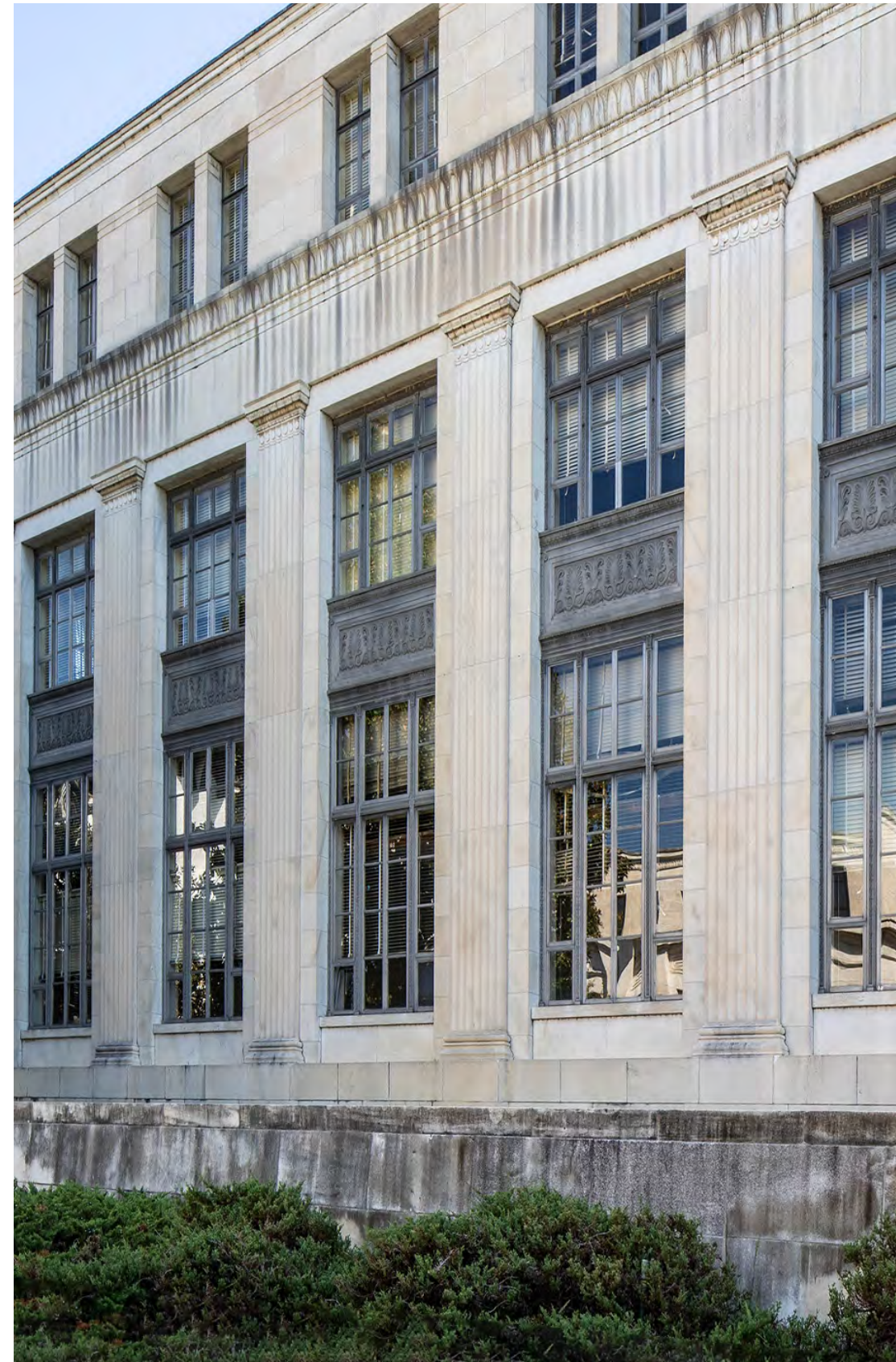
FRB-EAST EXISTING WINDOWS SET BACK 14" FROM FACE OF PILASTERS
