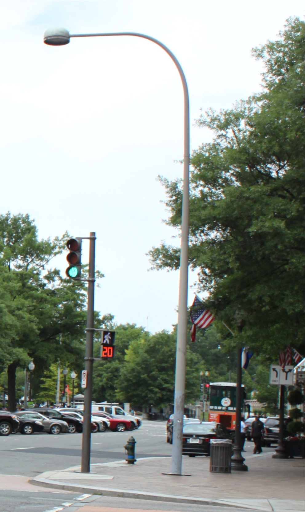
EXISTING ROADWAY COBRA POLES
