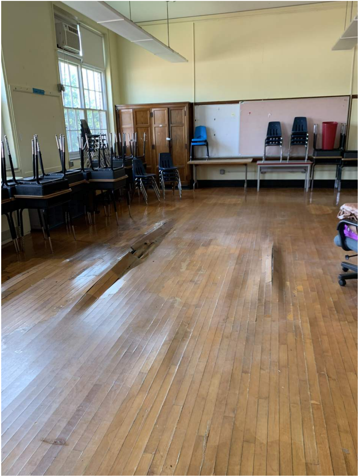
WARPED WOOD FLOORING IN CLASSROOM
