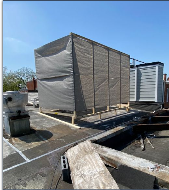
Upper Roof Unit
