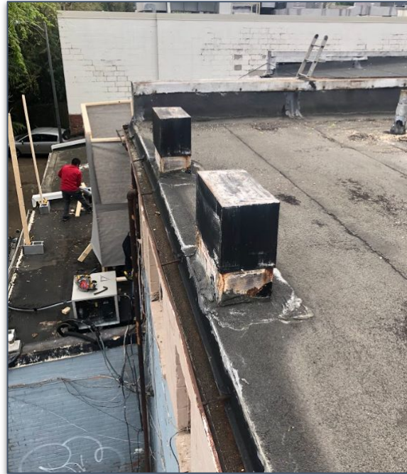
Lower Roof Unit
