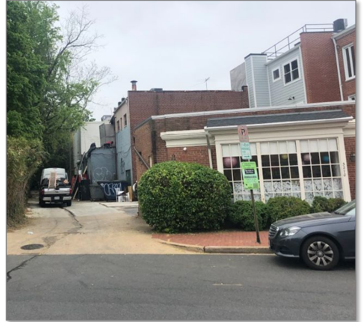
Facing South from North Side of S Street. Unscreened lower level unit and unscreened upper roof unit.
