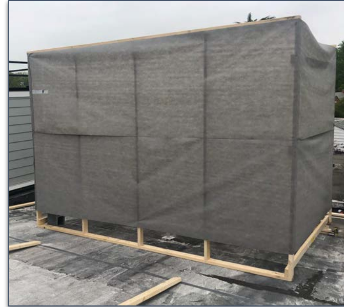
Upper Roof Unit
