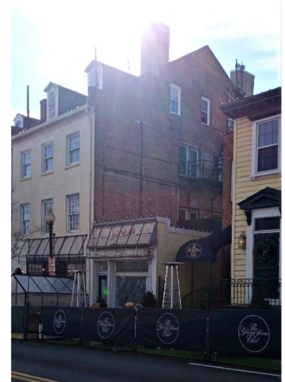
EXISTING BUILDING FRONT SIDE VIEW
