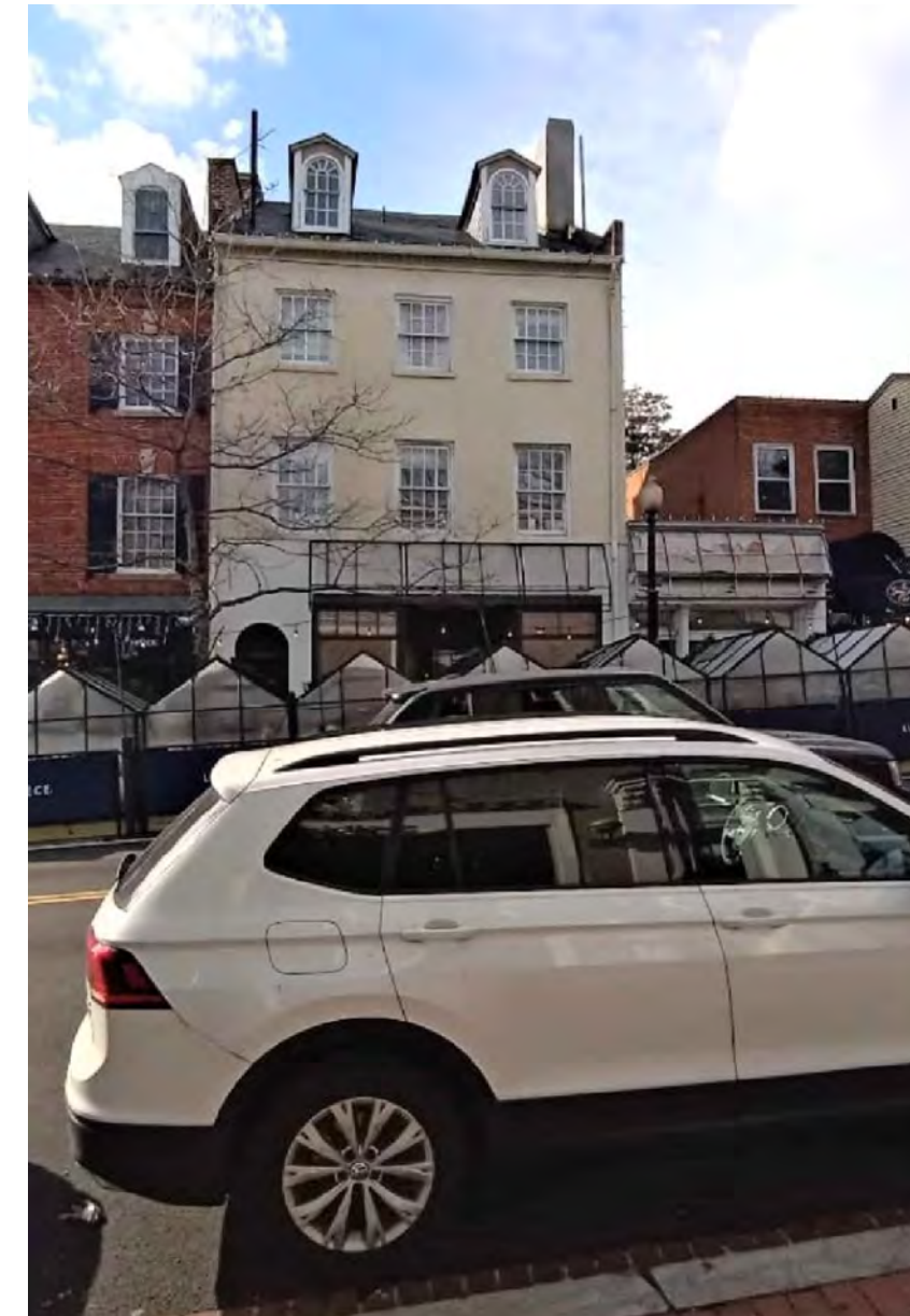
EXISTING BUILDING FRONT VIEW
