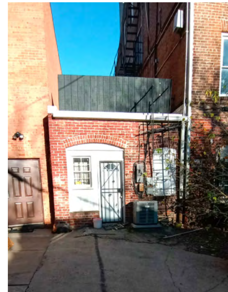
EXISTING BUILDING REAR VIEW
