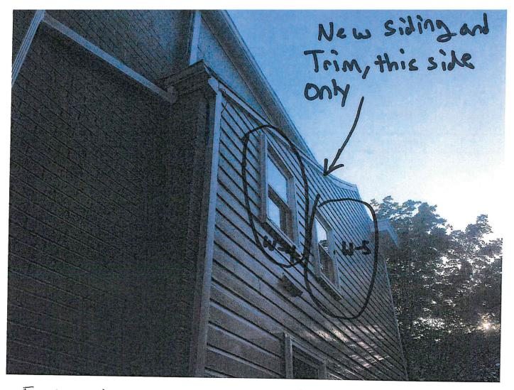
• Enstall 2 New Maruin All Wood DH 28×33<sup>3</sup>/4 windows with no grids. Full Jamb Install, we will Install new Brick mould and subsill to match existing. (W-4, W-5) Dostall new Dutch hap wood siding and new wood trim. Siding and trim protiles / sizes to Match existing. Left side of house only. Dutch lap is s".
