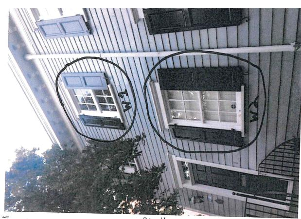
· Install new 28× 44314" Marvin All Wood DH with 6/6 Grids, Fullsamb Install, we will Install NEW Brickmould and subsill to match existing. Reuse Shutters (W-I)
