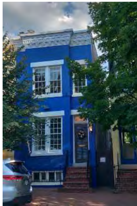
1 Street View of Building A01
