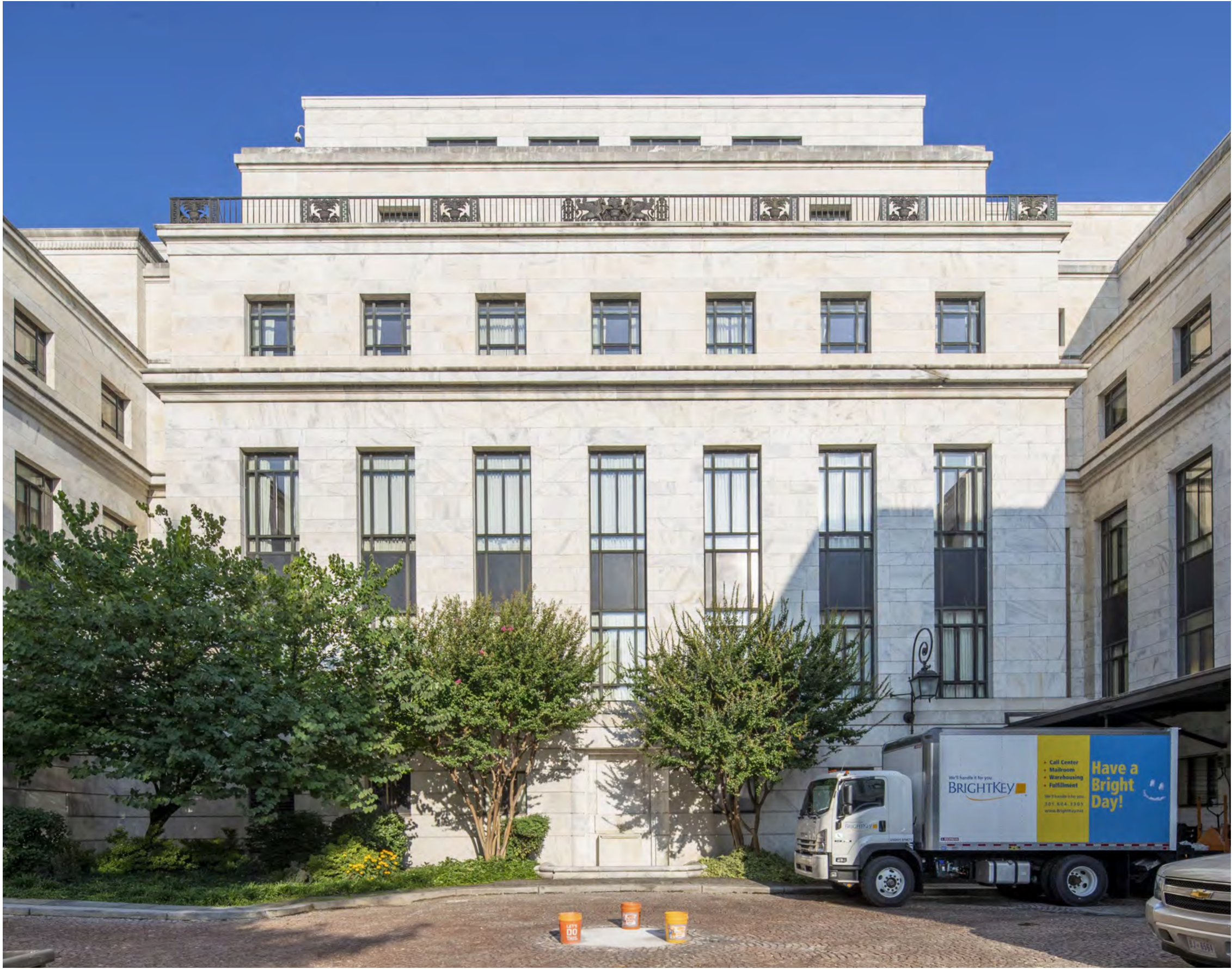
DOUBLE HEIGHT BRONZE WINDOWS W/ ALBERENE STONE SPANDREL PANELS
