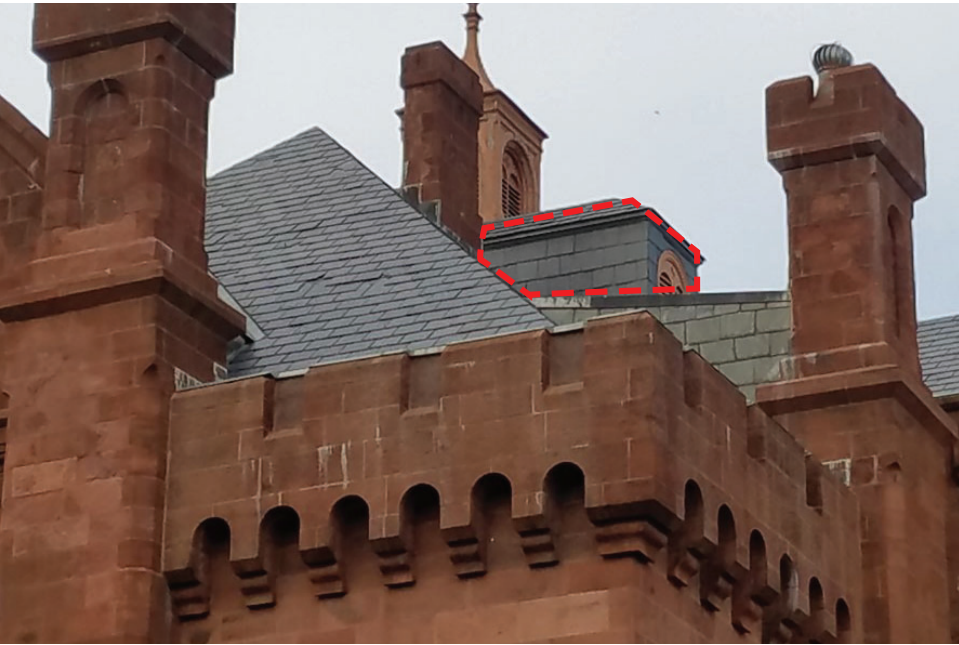
Figure 3.3.1.d - Image of southeast roof. Existing elevator penthouse to be removed(shown in dashed red lines).
