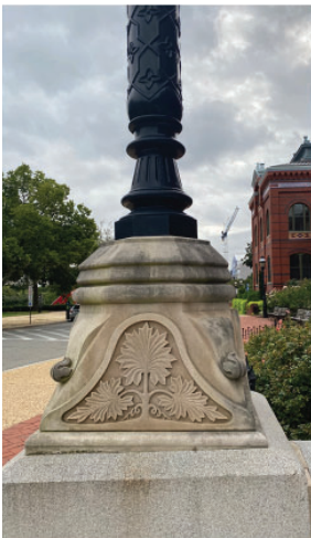
Figure 3.1.1.d - Image of cast stone lighting base at AIB.
