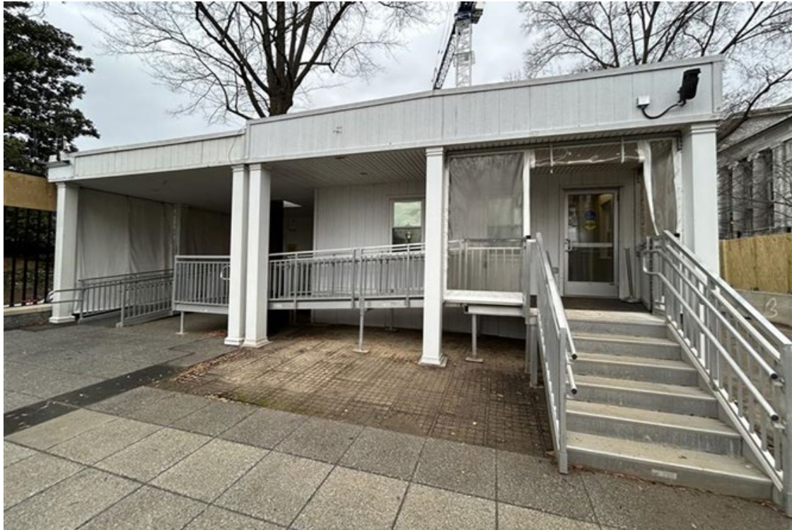
VIEW OF THE EXISTING VISITOR SCREENING TRAILER ENTRANCE ON EAST EXECUTIVE AVENUE.
