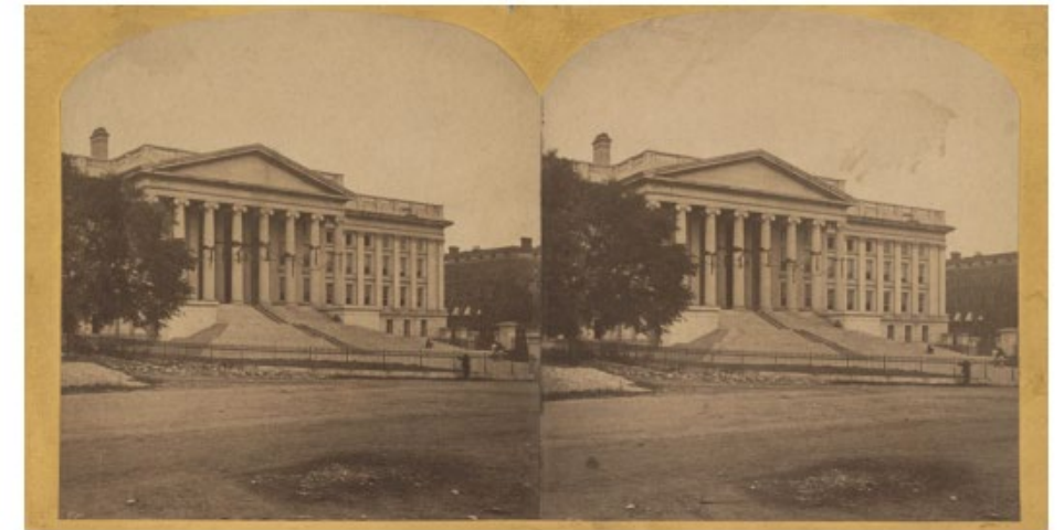
Figure 2-54. An 1865 image of the south facade of the Treasury Building following Lincoln's assassination. (Source: Library of Congress, https://www.loc.gov/item/2017645157/ , accessed January 2, 2024)
