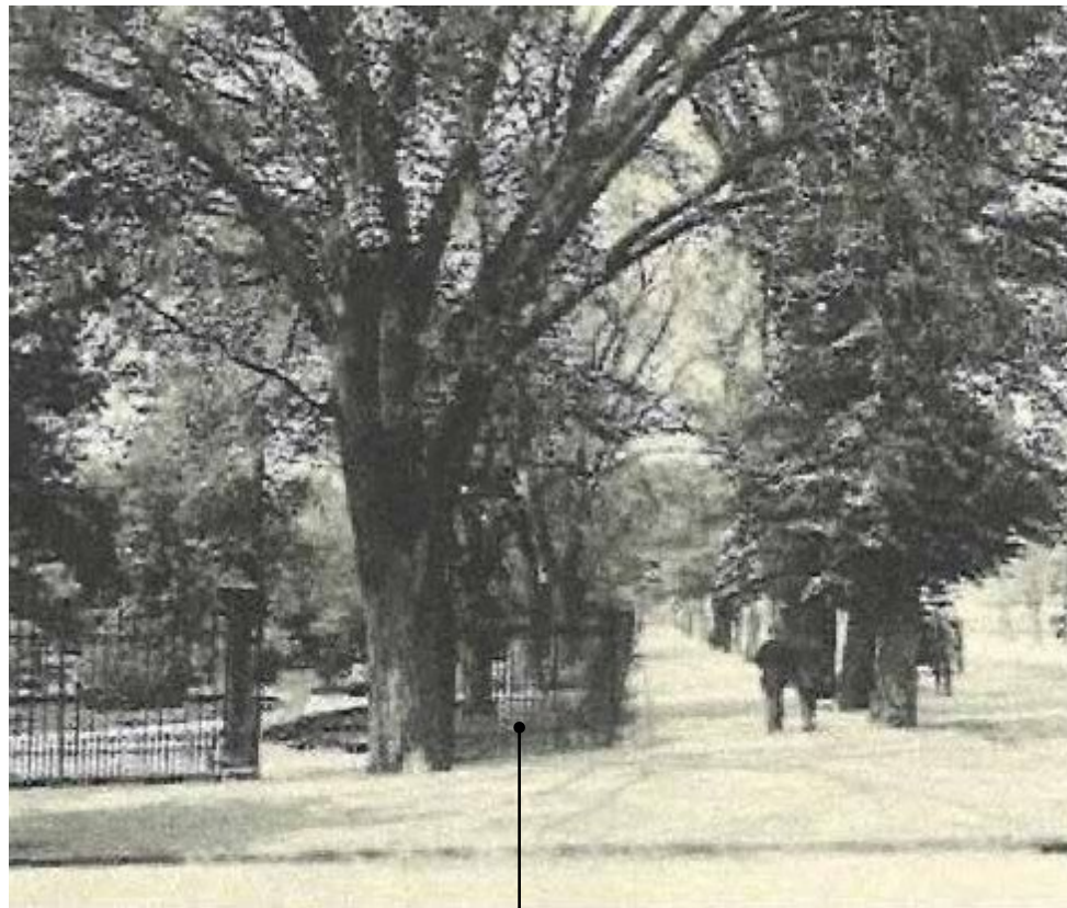
1880 H Street NW Looking west
