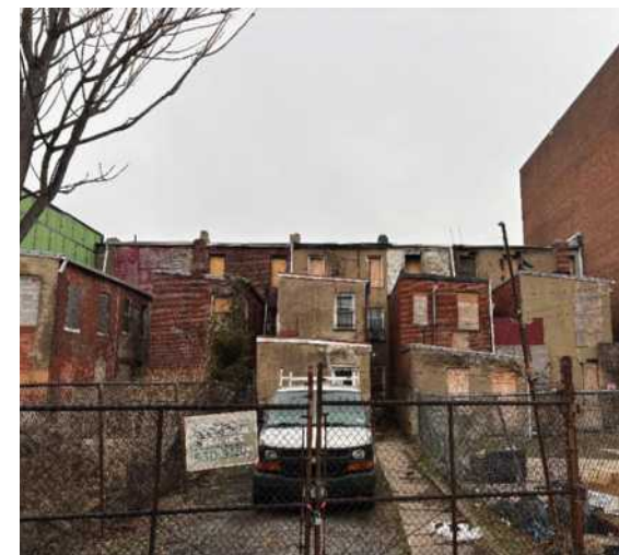
5 Rear of Adjacent Row Houses
