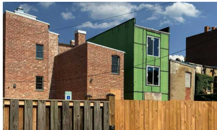
4 Rear of Adjacent Row Houses
