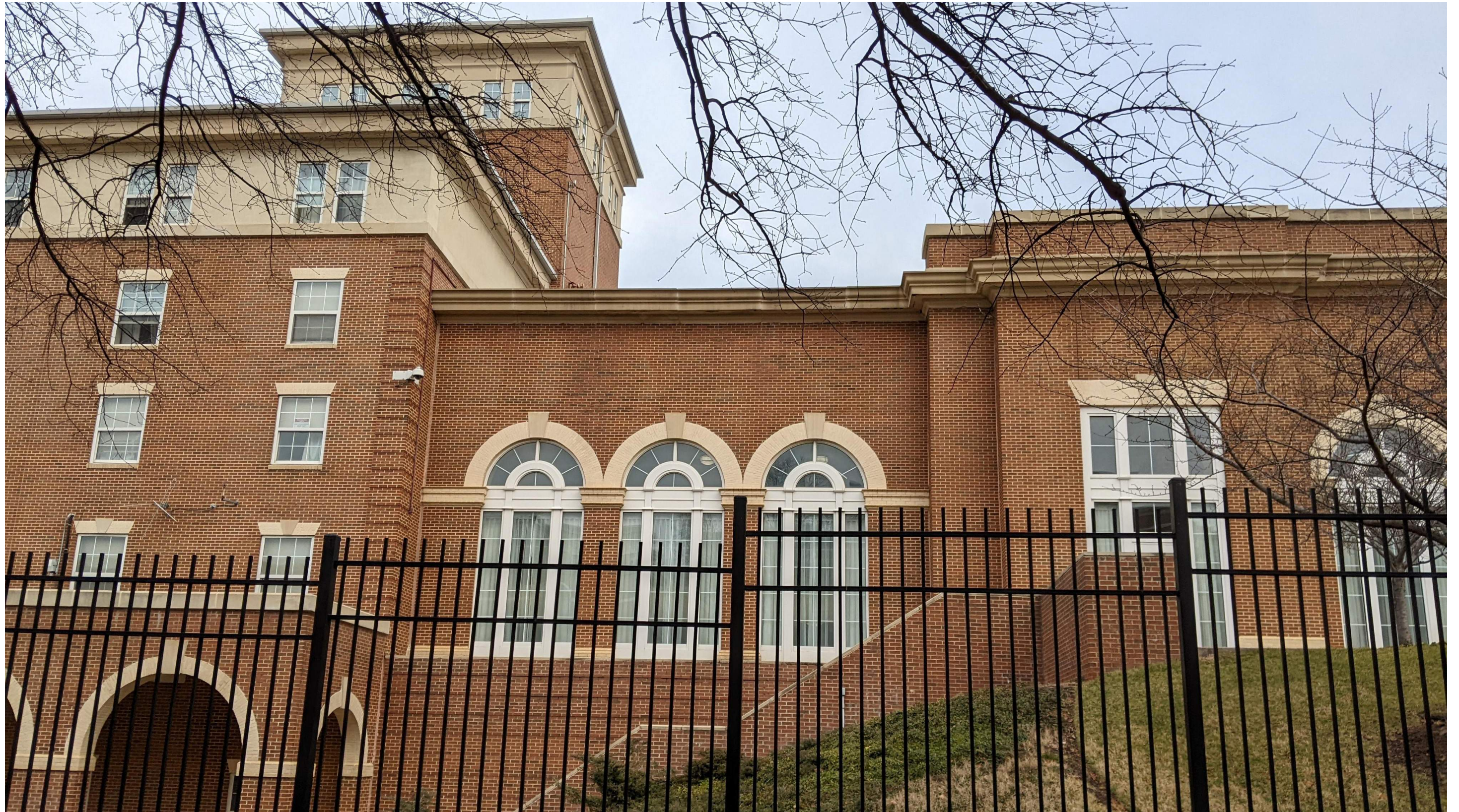
View of Building South Elevation from L Street
