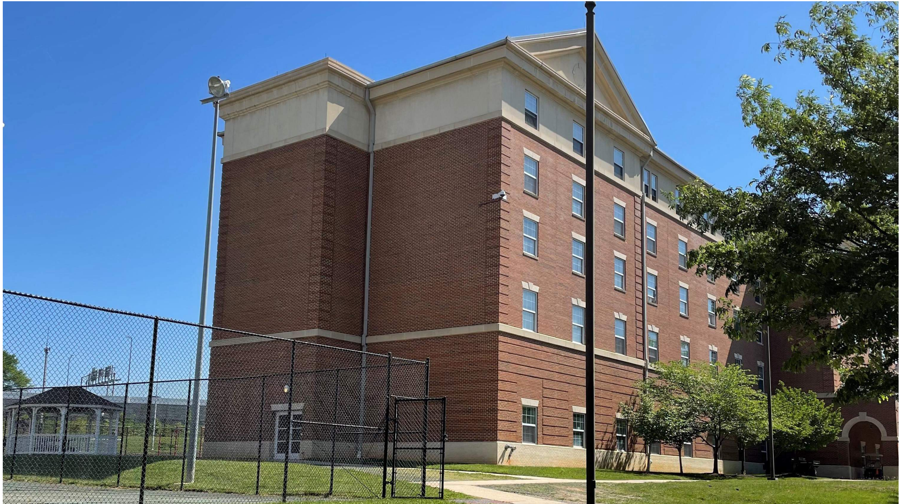
View of West End of Building 25 from L Street
