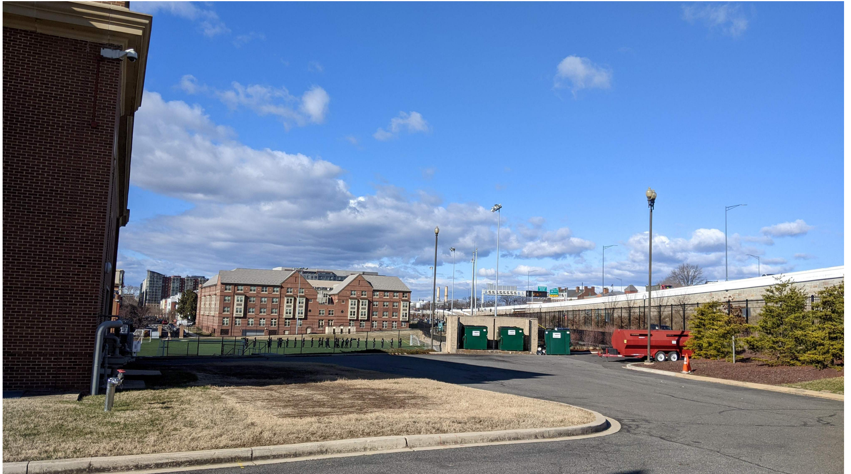
View of Building 25 Loading Dock Area and I-695 Beyond
