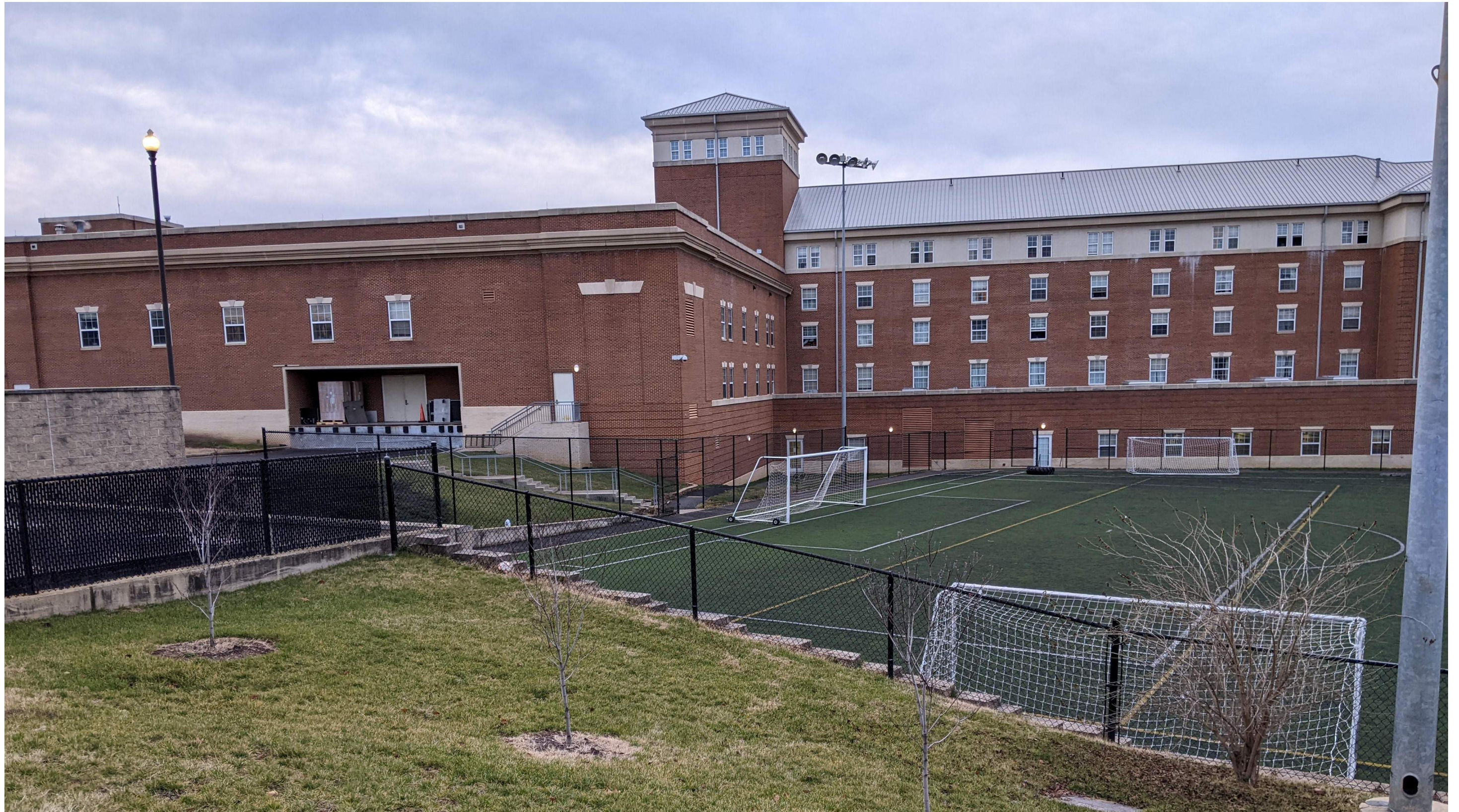
View of Building 25 Loading Dock Area and Stairway to Athletic Field
