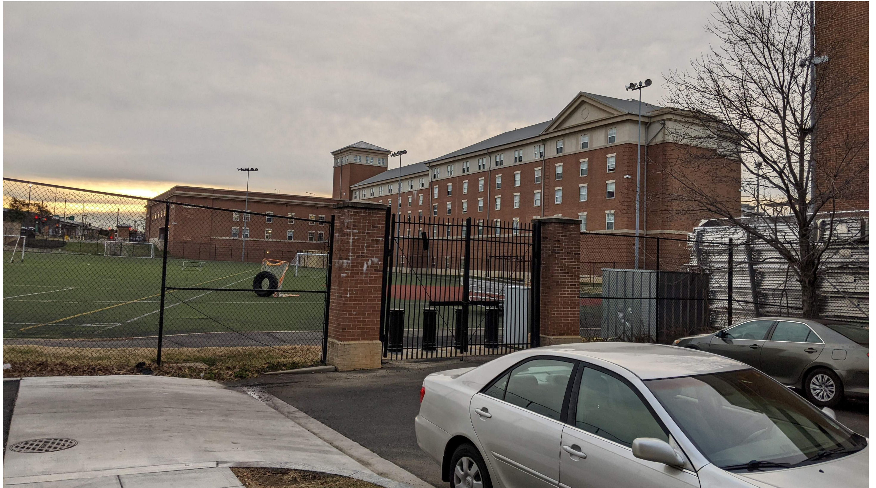
View of Building 25 from the K Street Security Gate
