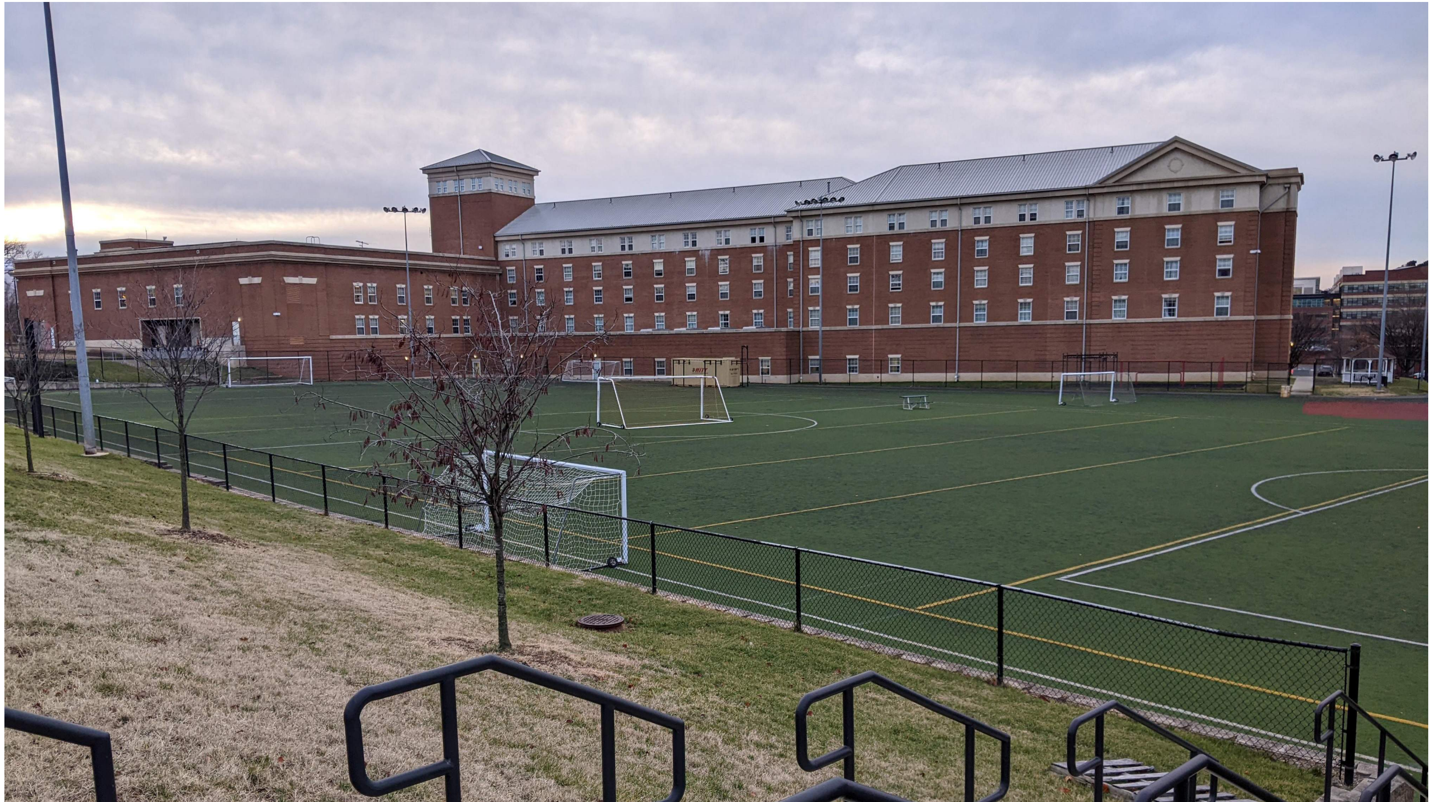
View of Building 25 from Virginia Avenue
