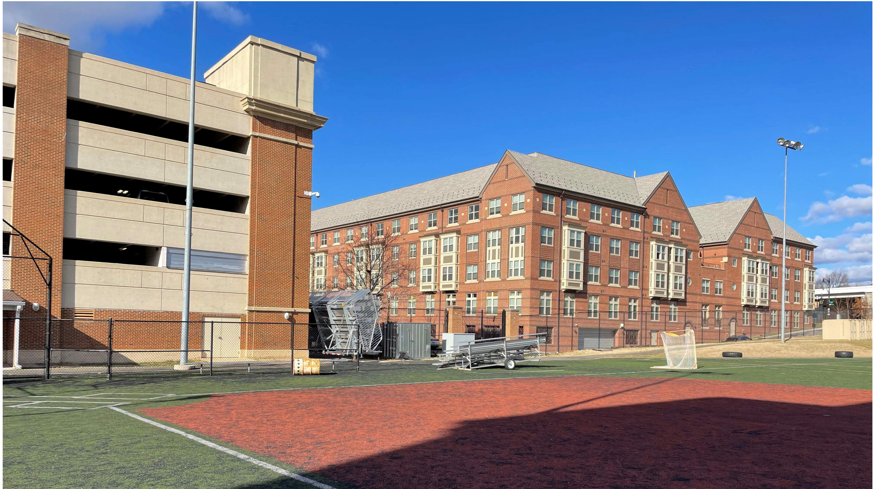
View of Building 26 Parking Garage and the K Street Entry Gate
