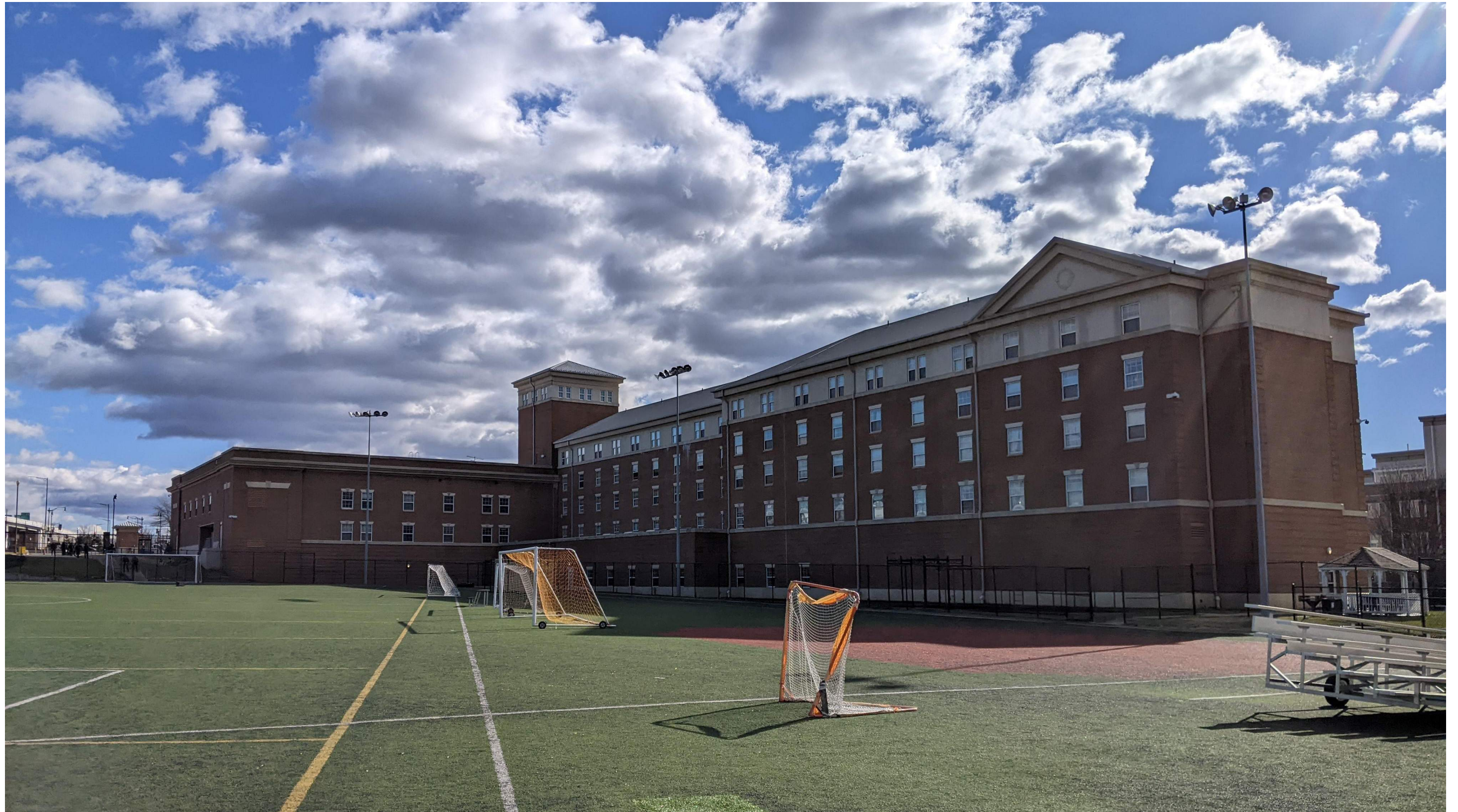
View of Building 25 from the Athletic Field
