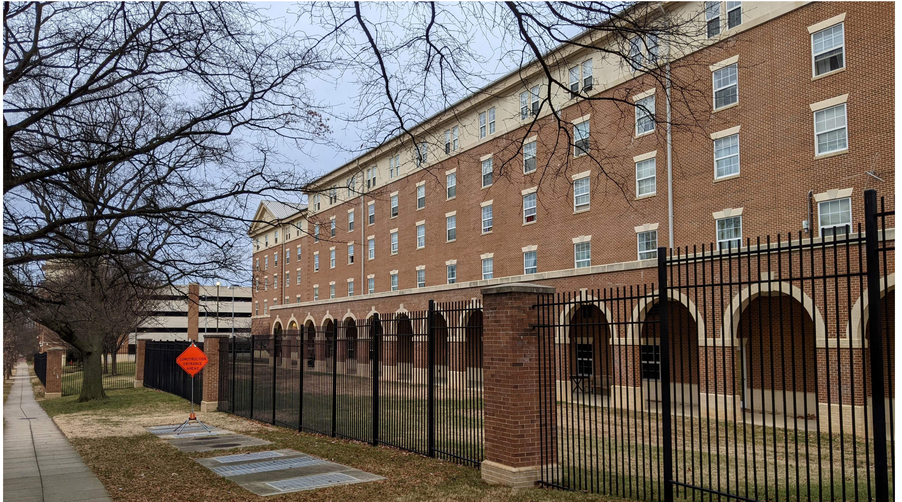
View of L Street Fencing and South Side Colonnade
