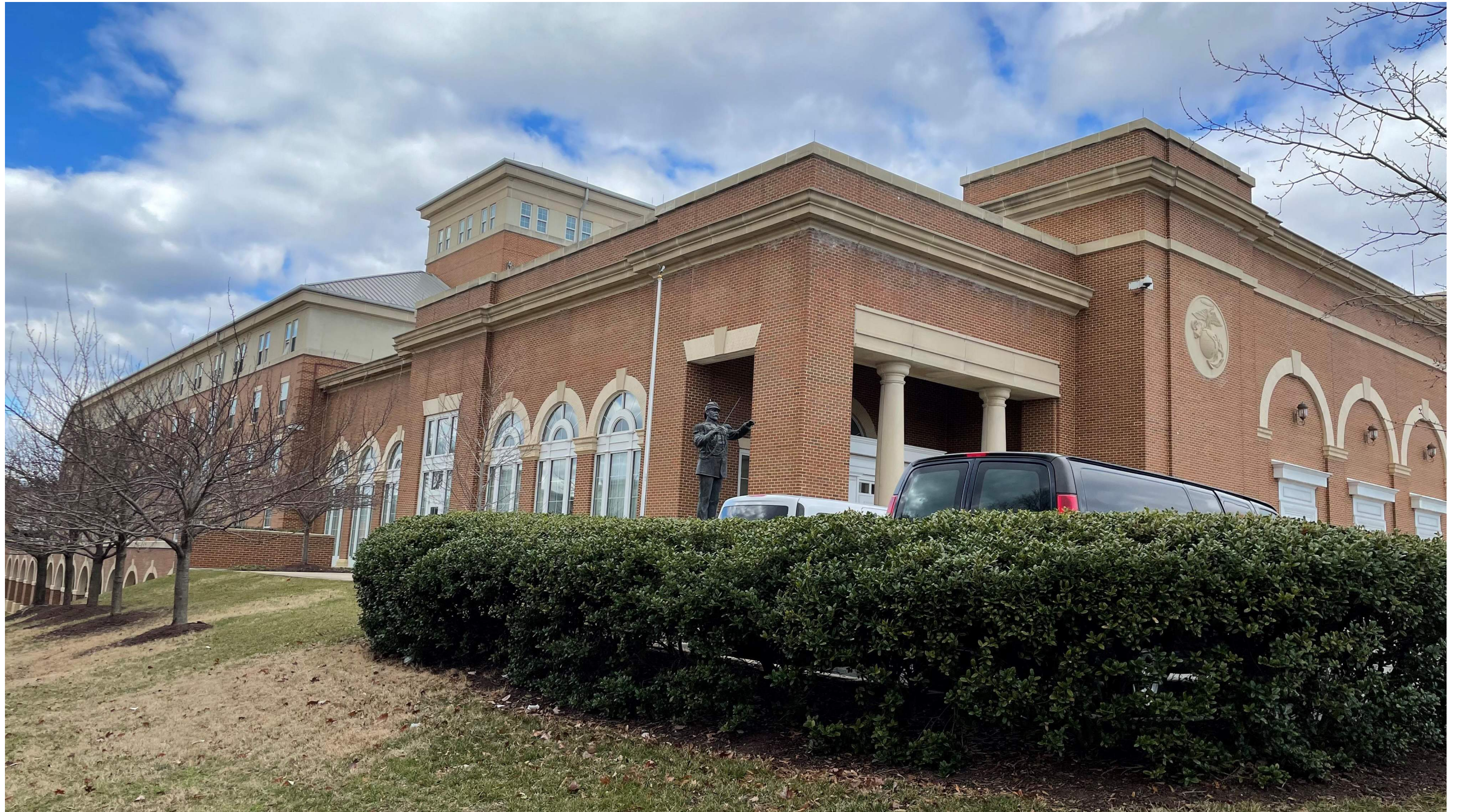
Detail View of Main Entrance to Building 25
