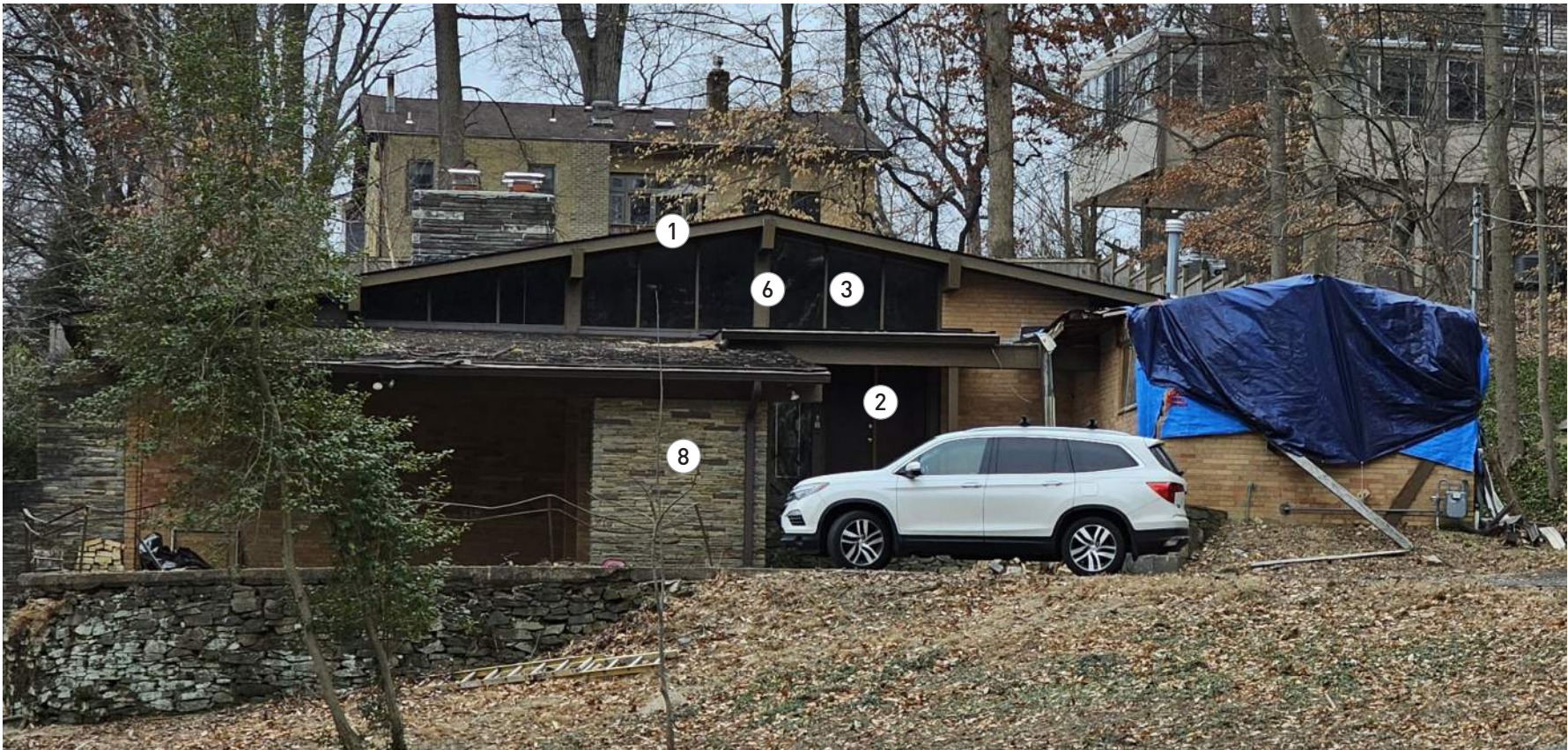
view from driveway (north elevation)
