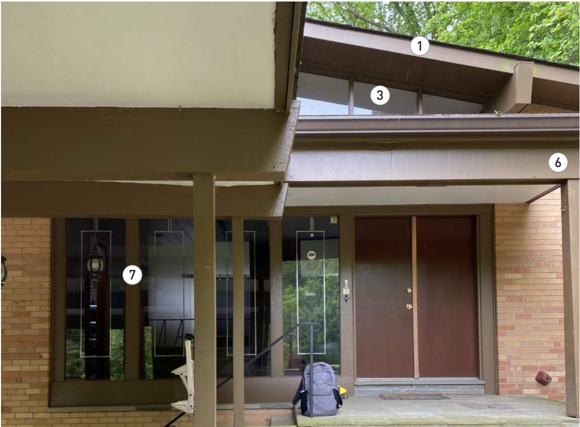
north elevation detail view
