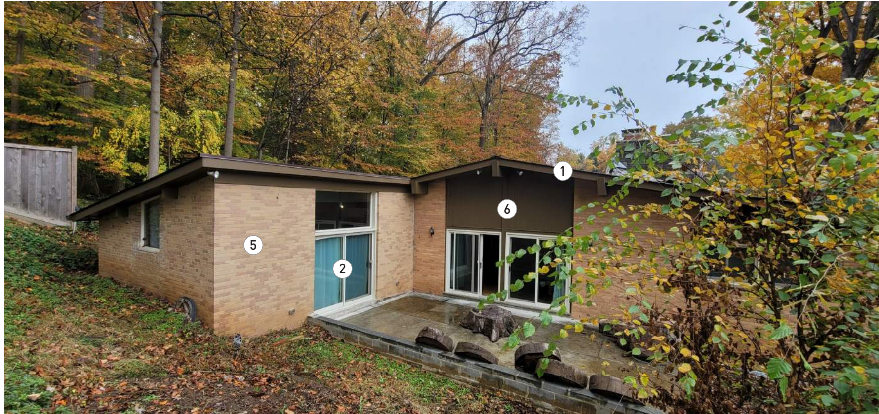
view from backyard (south elevation)
