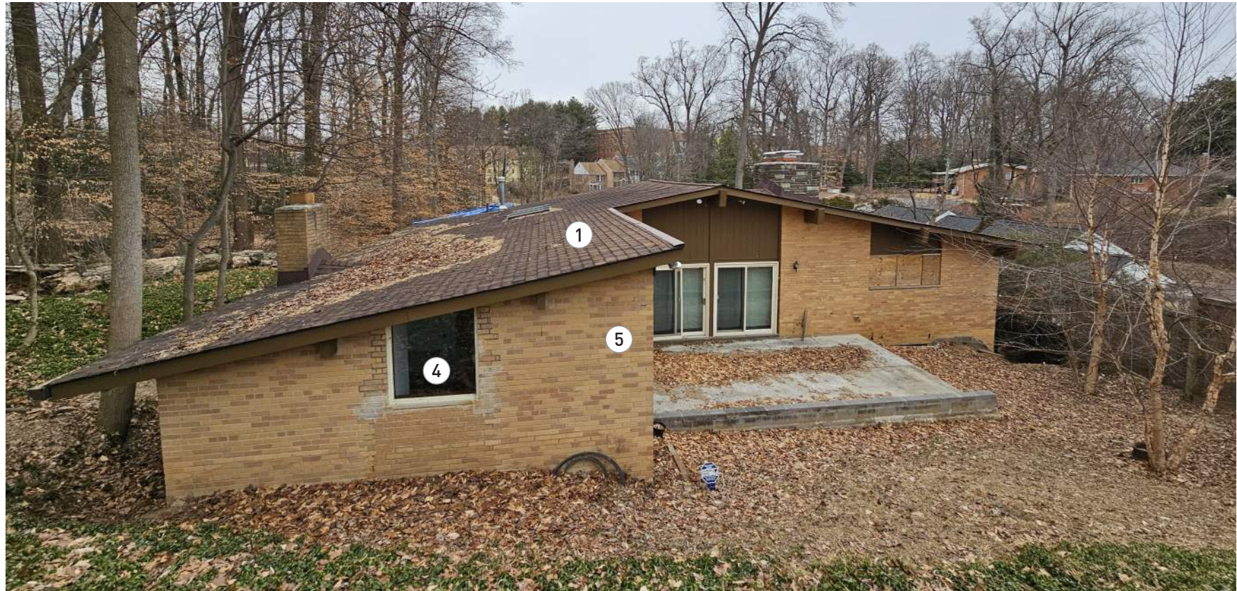
view from backyard (south elevation)
