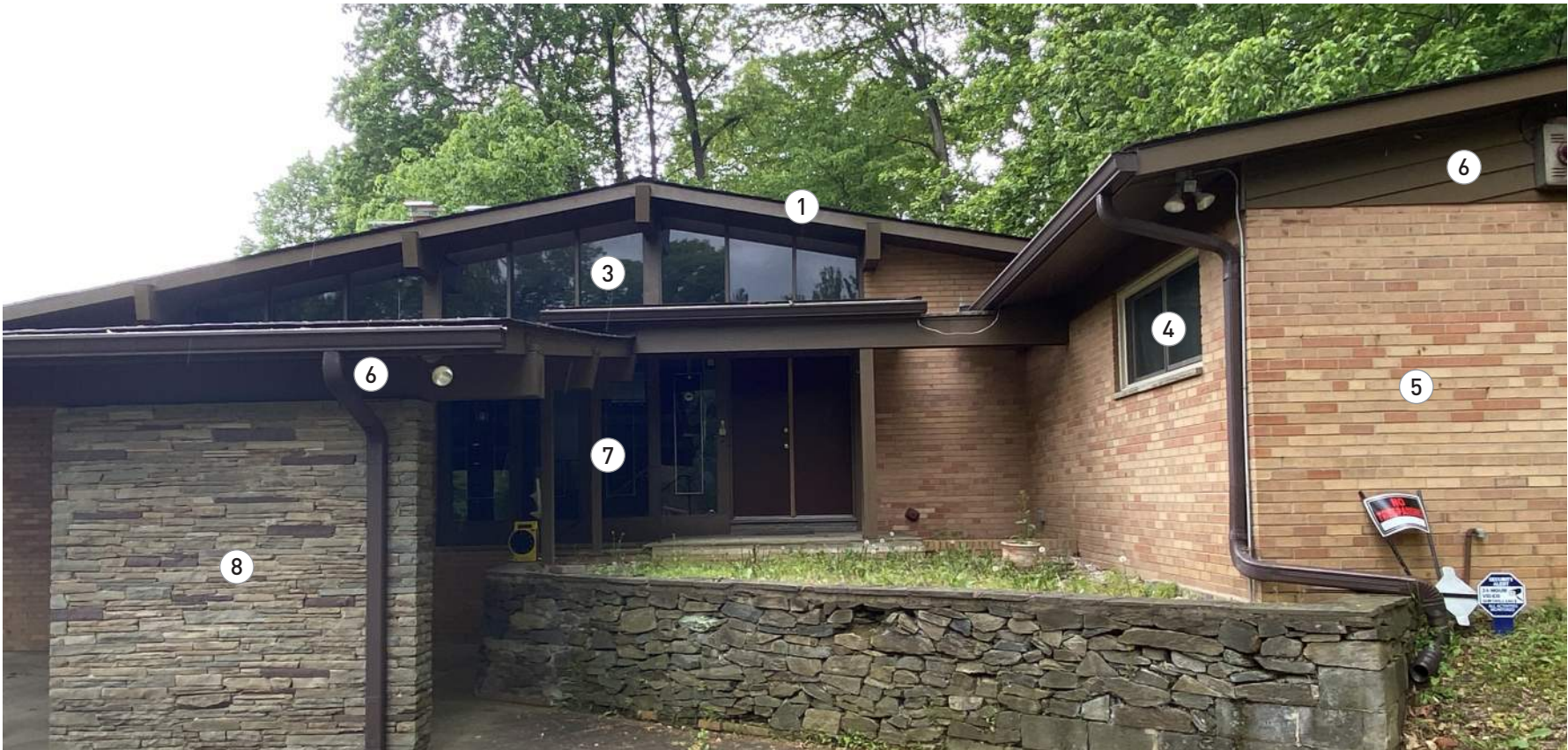
view from driveway (north elevation)
