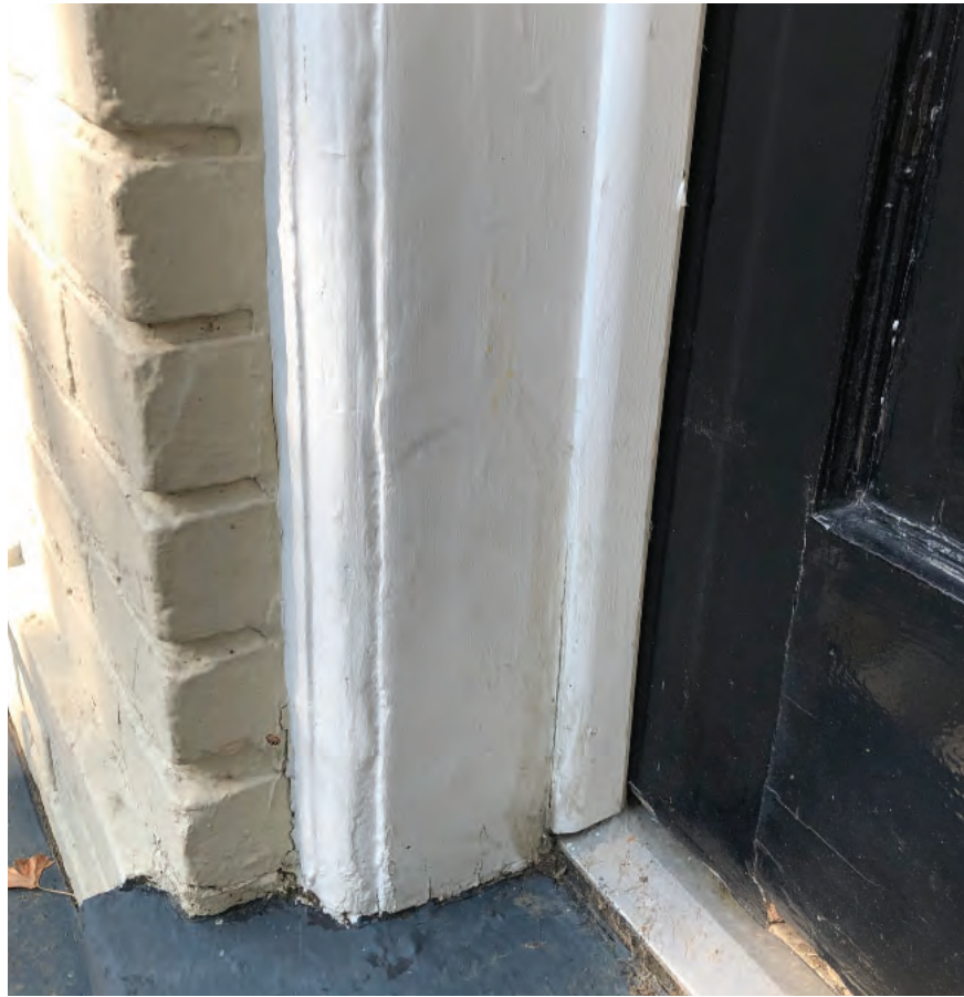
NEW BRICK MOLD & DOOR STOP TO MATCH EXISTING; TO BE CUSTOM MILLED WITH EXISTING TRIM AS A REFERENCE
