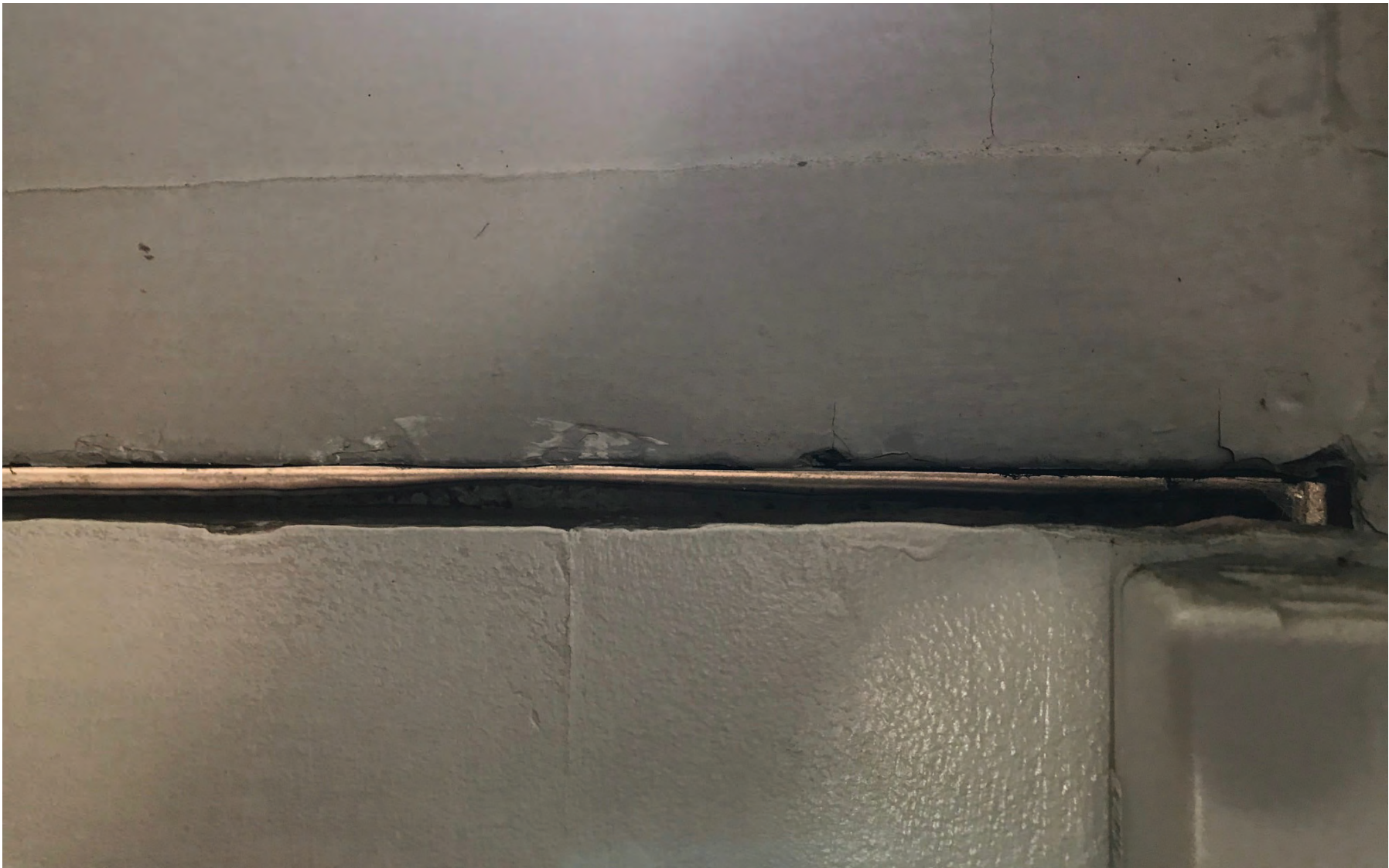
EXISTING DOOR CONDITION; DAYLIGHT VISIBLE AROUND TOP OF DOOR SLAB
