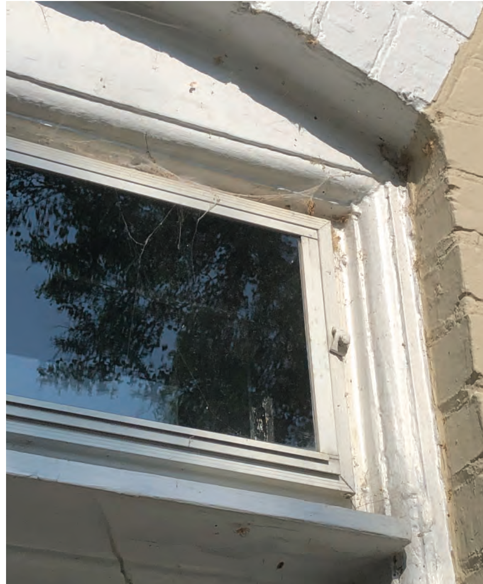
EXTERIOR STORM WINDOW & NON-HISTORIC TRIM BEHIND TO BE REMOVED
