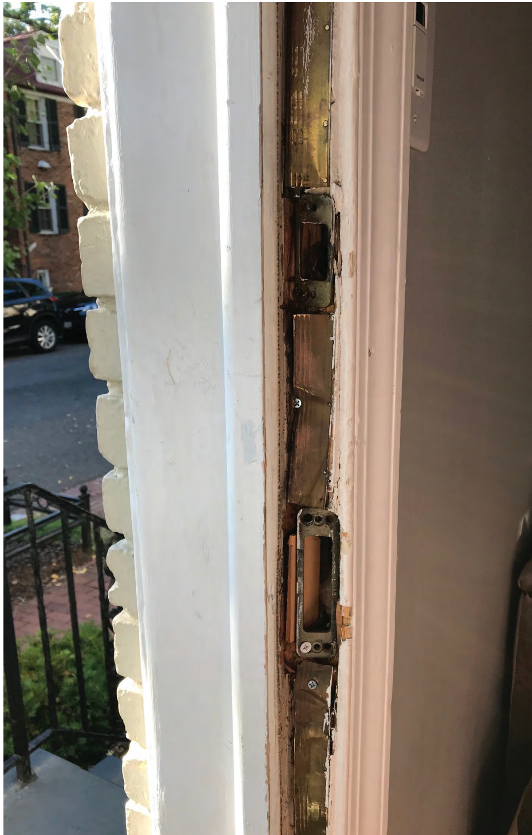
JAMB CONDITION AT STRIKE PLATE SIDE
