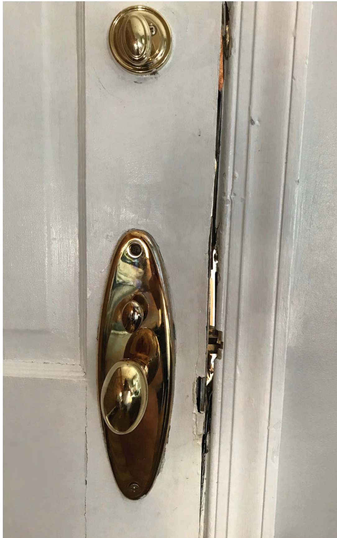
EXISTING DOOR CONDITION; DAYLIGHT VISIBLE AROUND SIDE OF DOOR SLAB
