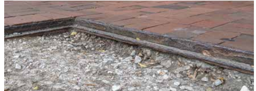
Typical compacted gravel in a treebox with resulting tripping hazard
