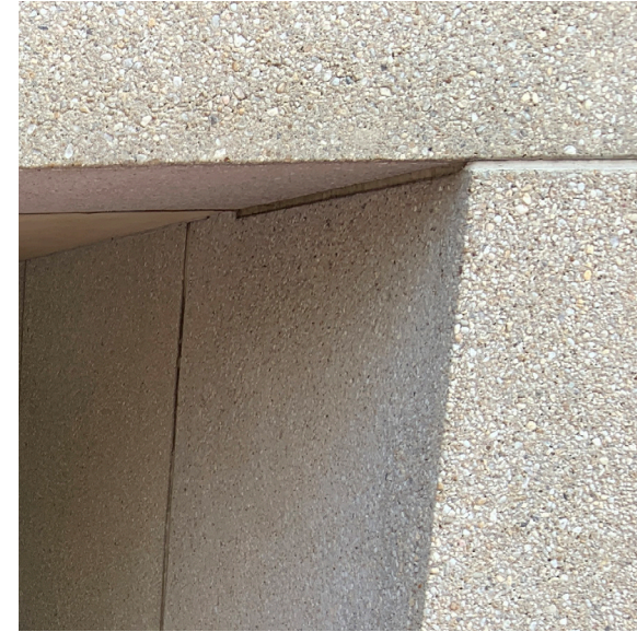
PRECAST CONCRETE [UDC CAMPUS]
