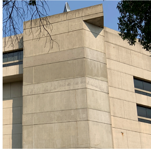
PRECAST CONCRETE [UDC CAMPUS]
