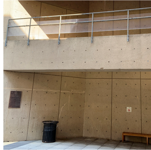
PRECAST CONCRETE [UDC CAMPUS]
