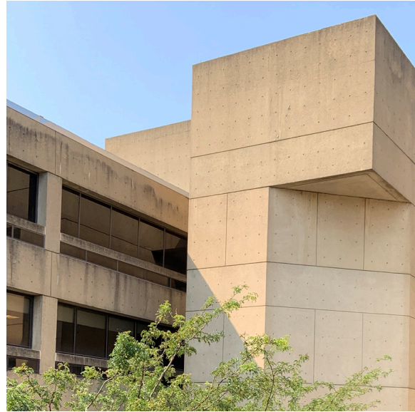
PRECAST CONCRETE [UDC CAMPUS]
