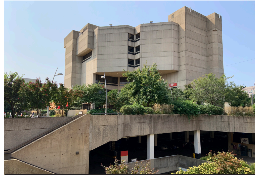
4 | View from Adjacent Building Looking SW
