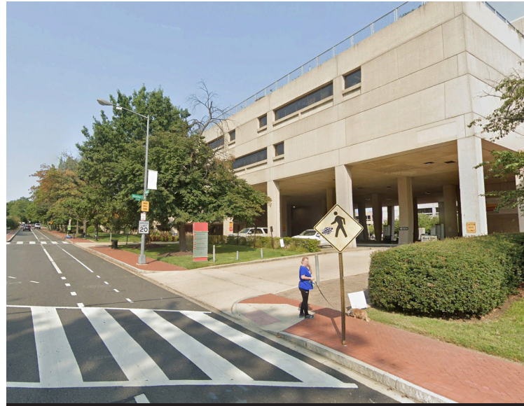
8 | View of Building 44
