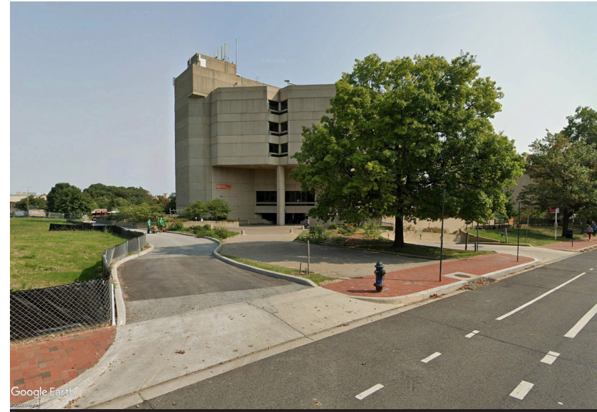
10 | View from Field Looking South
