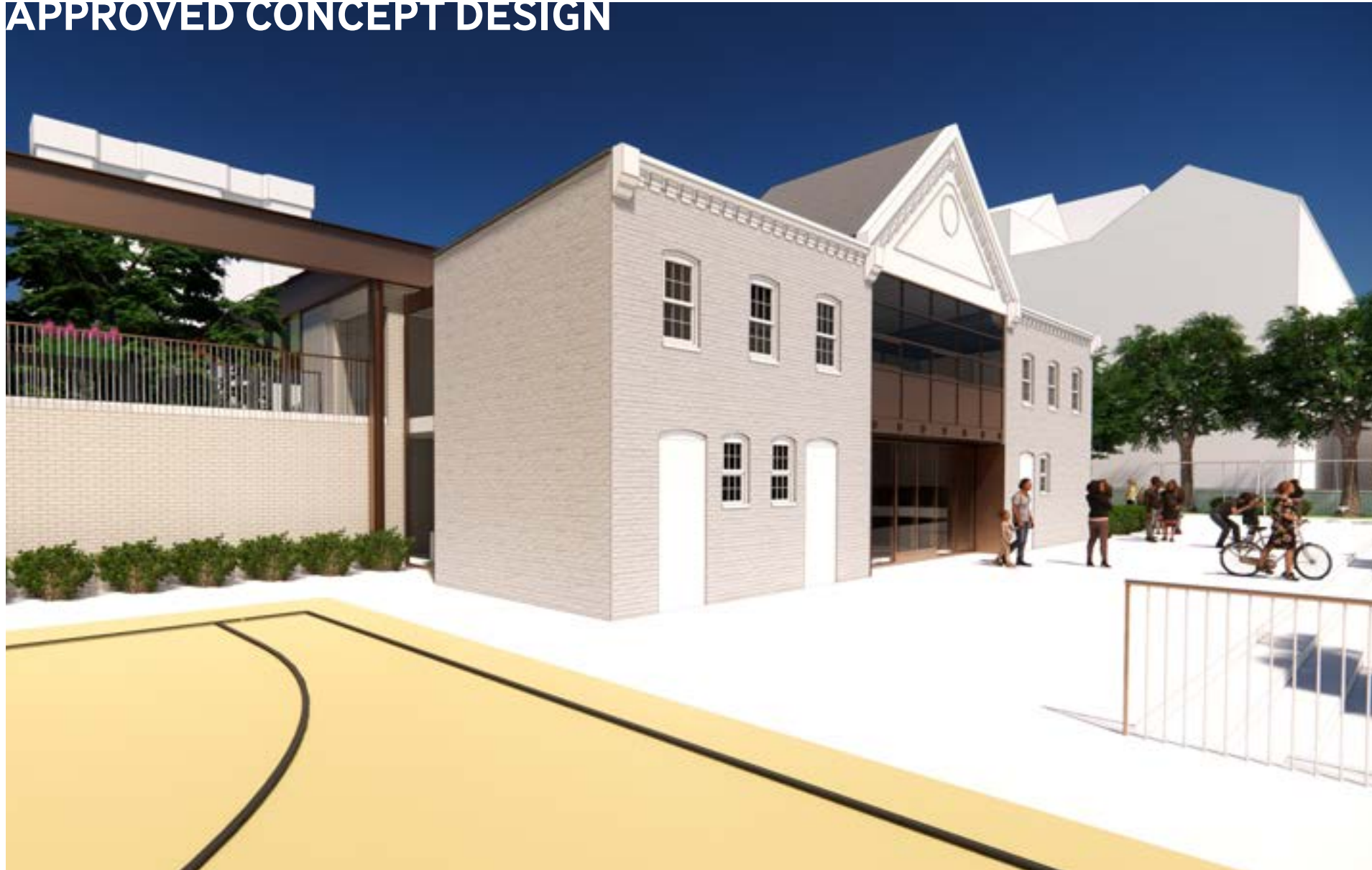
Existing Brick - Repointed, Restored, Repainted
