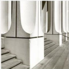
C.I.P. CONCRETE STRUCTURE
