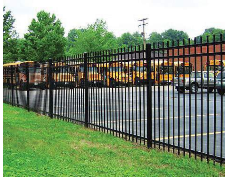
6 FT PERIMETER FENCE
