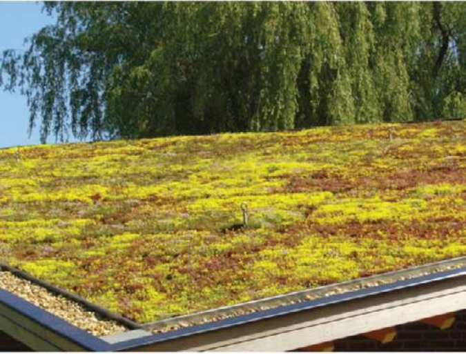
Green Roof Sedum
