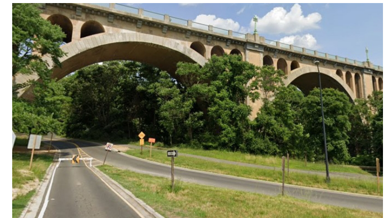
Under Bridge View from Rock Creek Park
