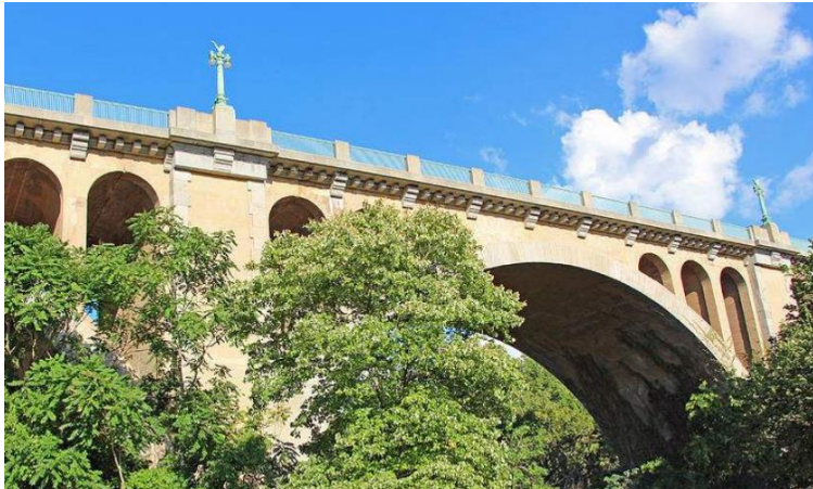
Under Bridge View – Rock Creek Park
