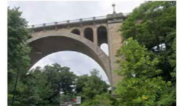
1995 Rehab of Connecticut Ave
