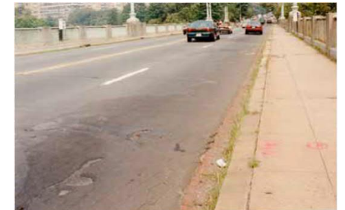
Bridge before 1995 renovation DDOT Historic Collections
