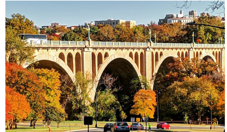
Bridge View from Rock Creek Park
