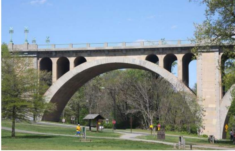
Under Bridge View - Rock Creek Park
