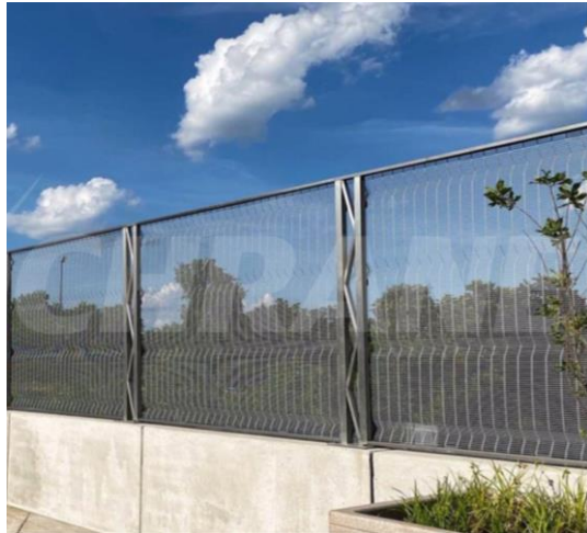
Reference Photo of Bridge 341
