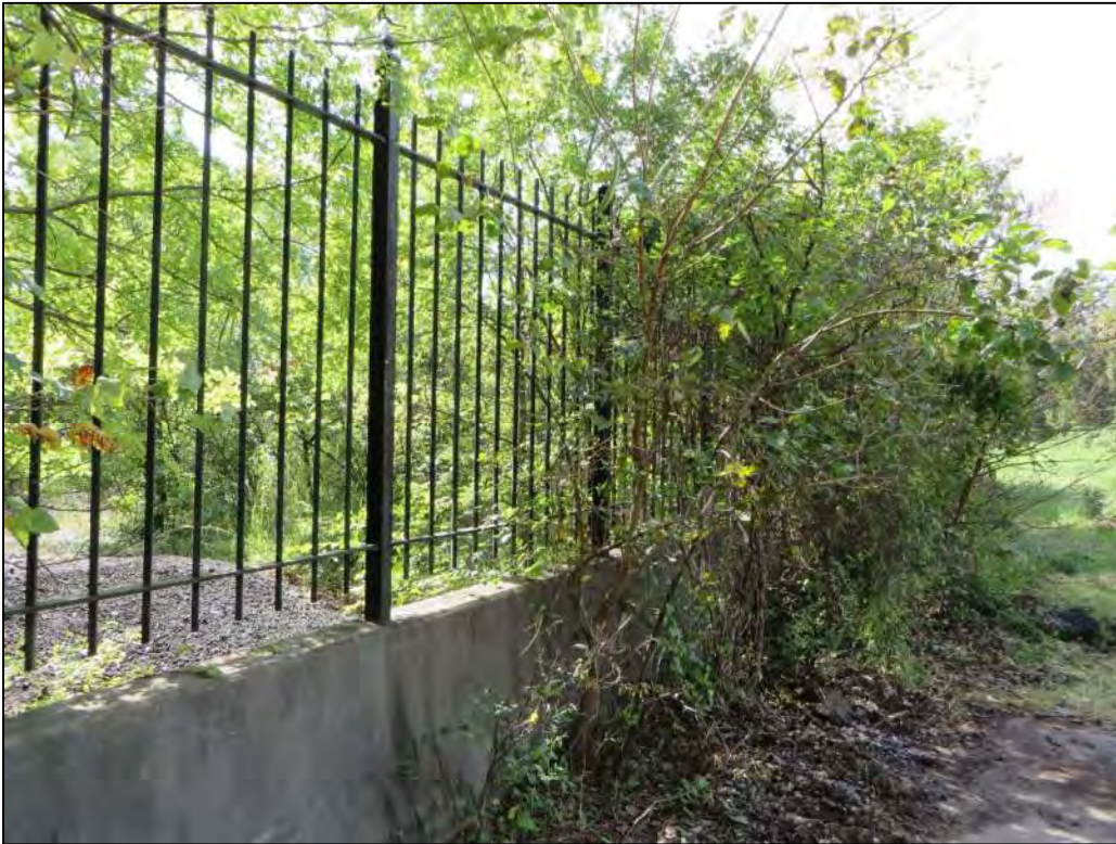
Figure 5 – Fence Type A, showing concrete foundation
