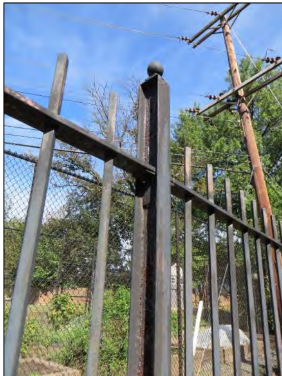
Figure 4 – Fence Type A, showing I-beam post and ball finial
