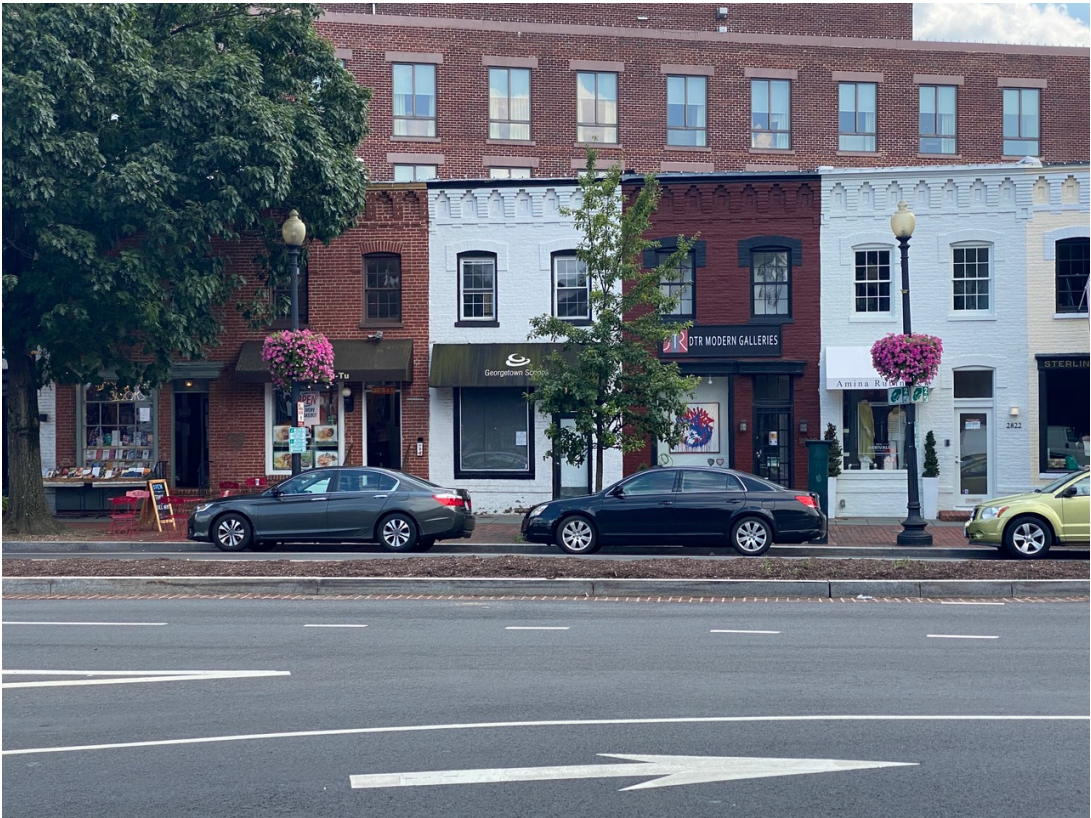
STREET FACADE (FROM ACROSS THE STREET)
