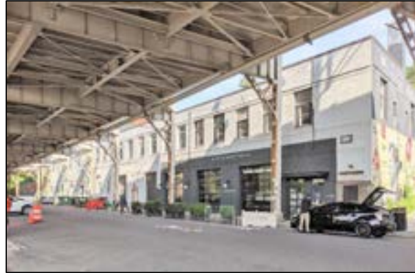
Figure 1. View of 3401 Water Street, NW from Water Street (EHT Traceries, September 2021)
