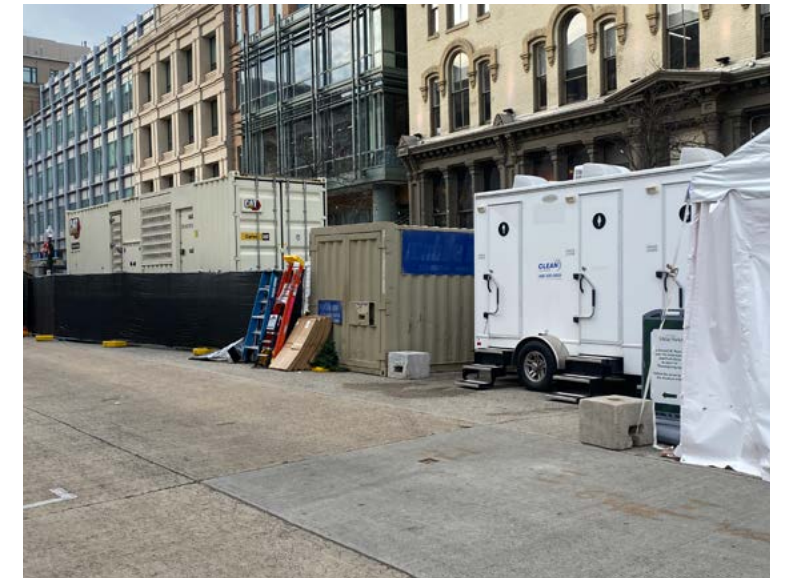
Temporary infrastructure elements for events
