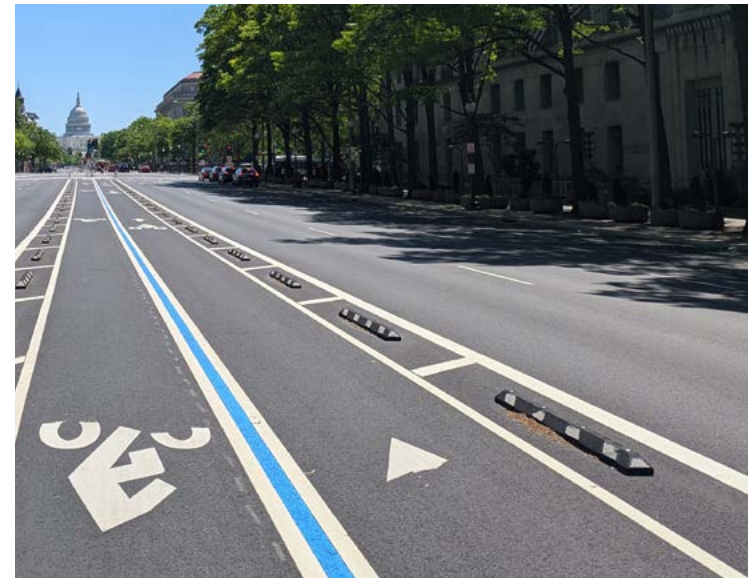
Lane dividers (or “caterpillars”), traffic signals, and other elements in the vehicular cartway
