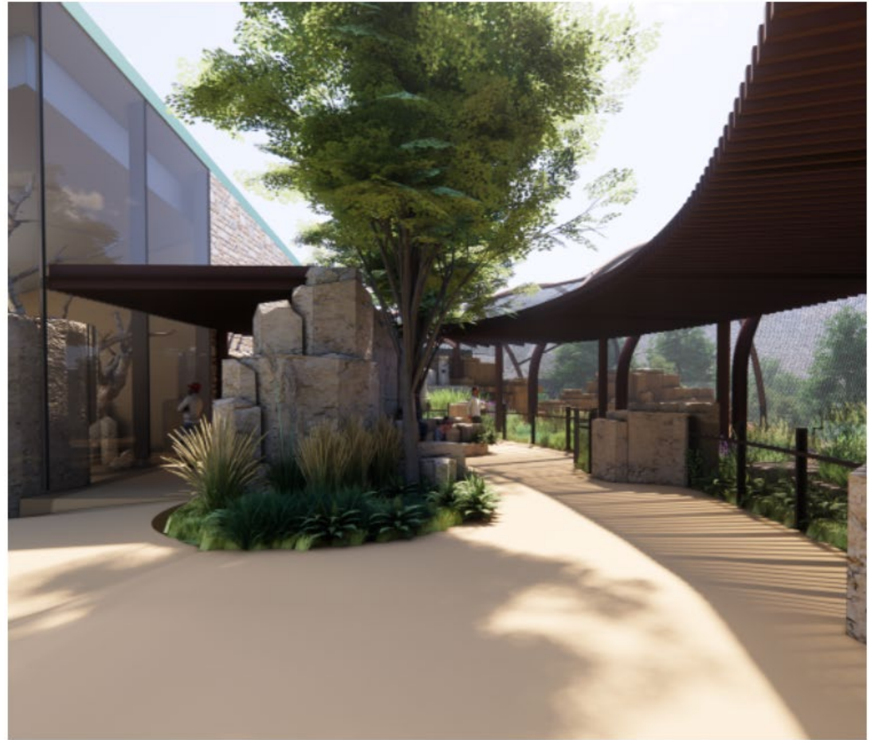
Figure 5.4.1.2: Revised Shade Structure at Central Plaza - Painted Steel Supports Separated from Painted Steel Arch Supports at Enclosure
