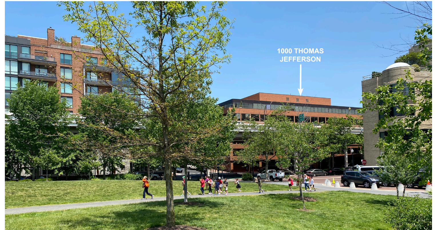
VIEWED FROM SOUTH WEST - 2
