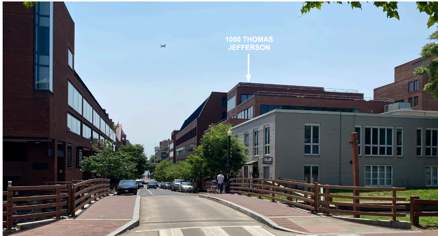
THOMAS JEFFERSON CANAL BRIDGE - 1
