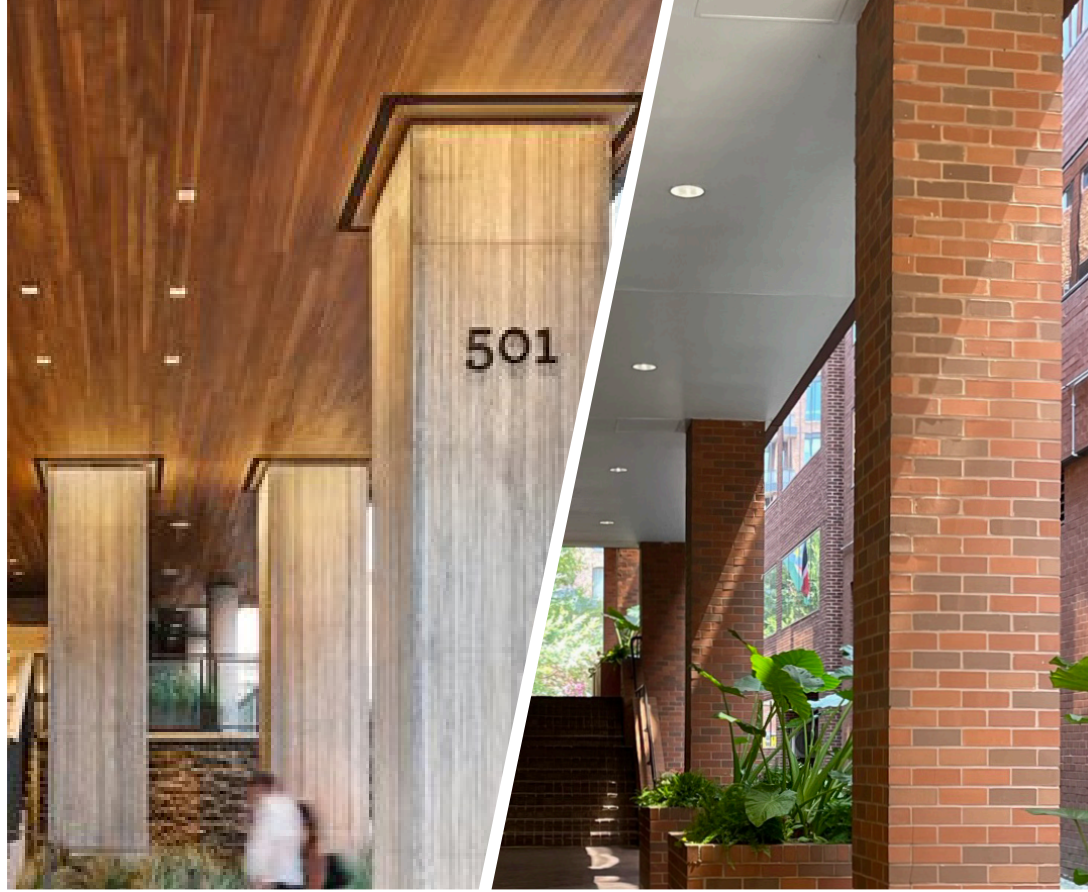
WRAPPED CEILING & COLUMNS
