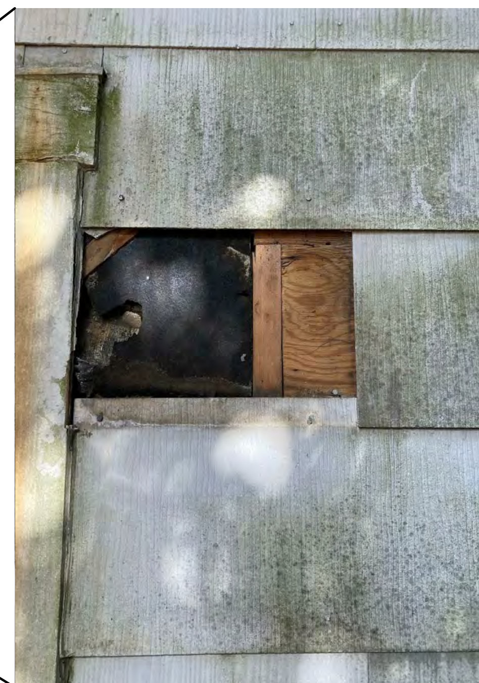
FIBER CEMENT SIDING TO BE REPLACED
