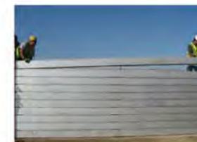
Install planks from above
