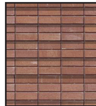
HORIZONTAL STACK BOND BRICK + ARTICULATION
