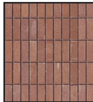
VERTICAL STACK BOND BRICK
