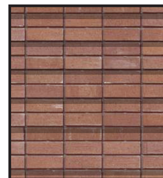
HORIZONTAL STACK BOND BRICK + ARTICULATION
