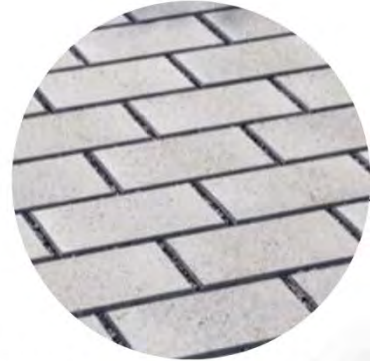
PERMEABLE CONCRETE PAVERS (PARKING SPACES)
