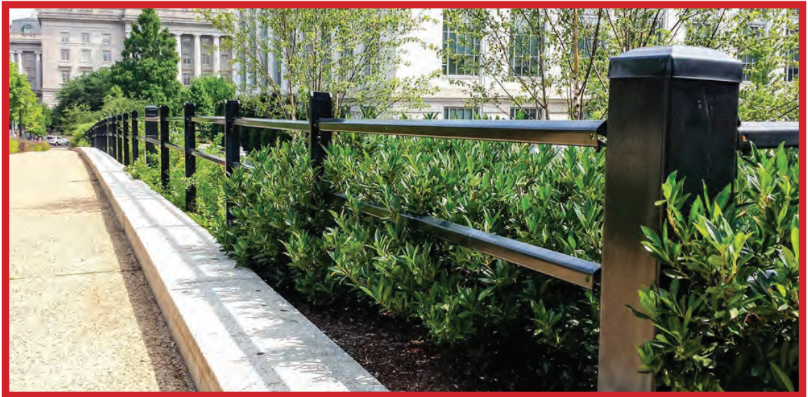
Cable Reinforced Fence System (installation) - National Museum of Natural History
